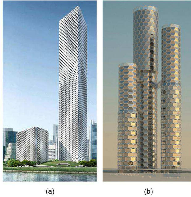
Figure 5-1 Examples of Hexagrid building a) Sinosteel building, (from www.i-mad.com ); b) Nanotower (from www.archicentral.com )
