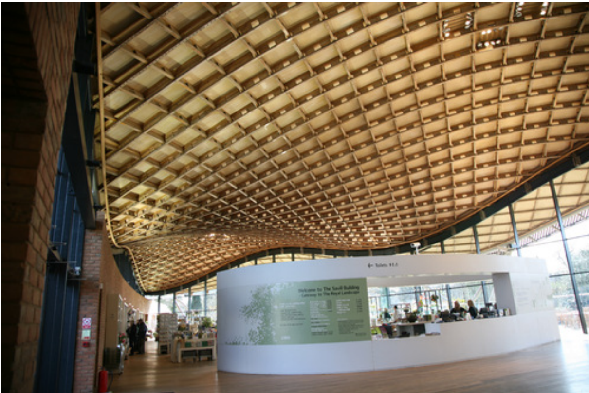
Figura 48 - La gridshell del Savill Building a Windsor (Glenn Howells Architects, 2006)
