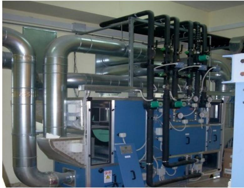
Figure 1.6: The desiccant-based AHU.
