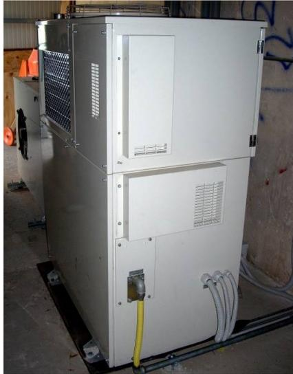
**Figure 1.9: The microcogenerator.**
