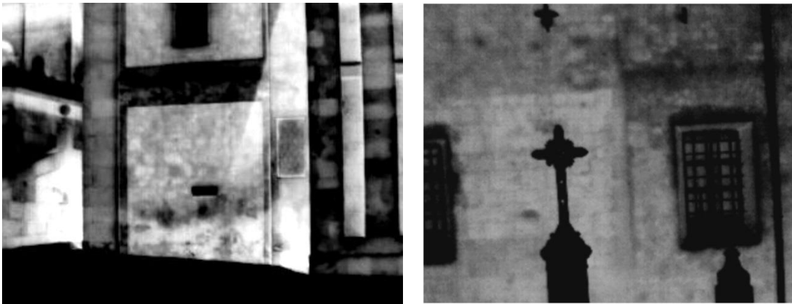
Figure A.8. Results of thermography
