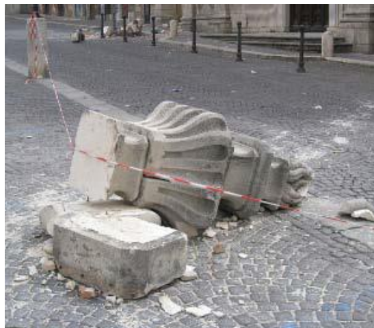
Figure 4.6. Damage class R.c - Overturning of self-standing elements (photo by [32])
