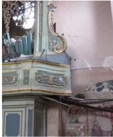
Figure 4.5. Damage class R.b - Unthreading and failure of connection. (photo by [32])
