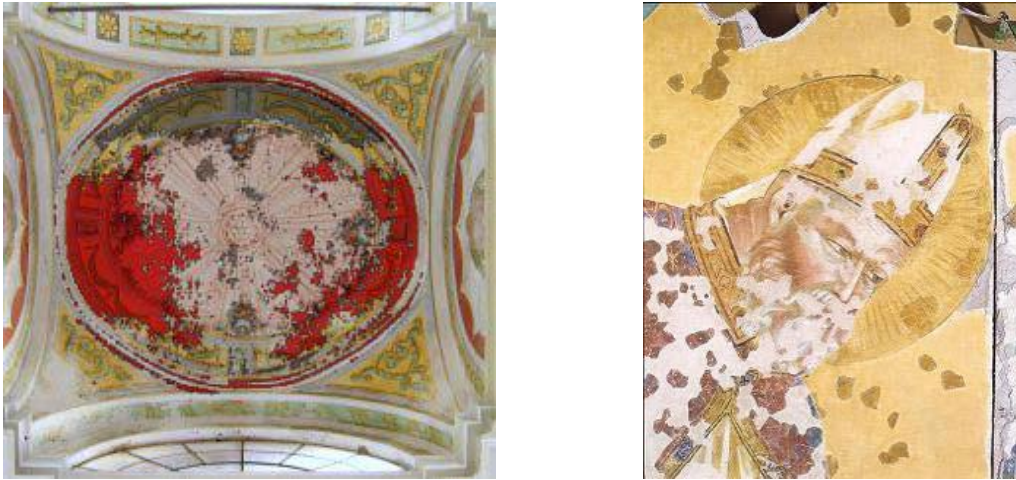
Figure 4.1. Damage class Q.a - Detachment of mural paintings (photo by [32])
