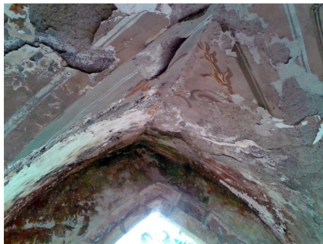
Figure 5.2. East walkway: presence of autotrophic organisms in the vault (photos October 11, 2013)
