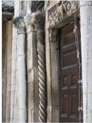
Figure 4.3. Damage class Q.c - Irreversible deformation (photo by [32])
