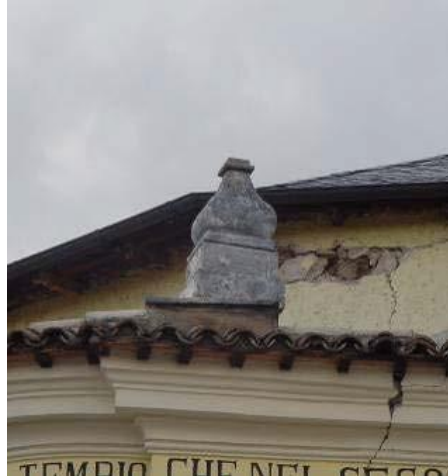
Figure 4.4. Damage class R.a - Dislocations (photo by [32])
