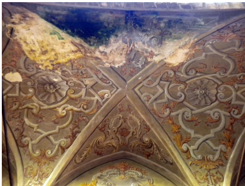
Figure 5.3. South walkway: presence of autotrophic organisms and detachments of intonachino in vault (photo February 1, 2013)
