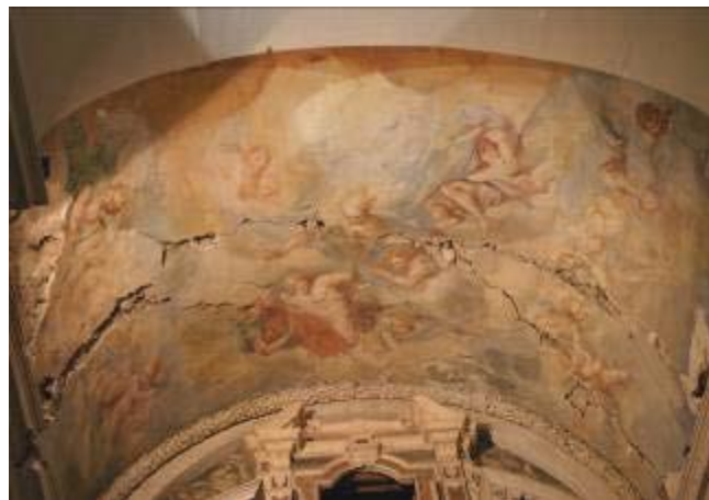
Figure 4.2. Damage class Q.b - Cracking (photo by [32])
