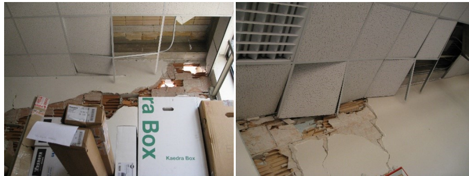
Fig. 2.25: Damage to suspended acoustic lay-in tile ceilings, 2009 Abruzzo Earthquake, L'Aquila, Italy
