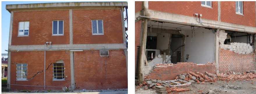
Fig. 2.6: Masonry infill walls in a reinforced concrete frame
