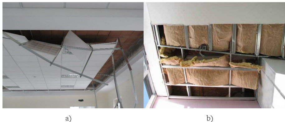
Fig. 2.23: Damage to suspended lightweight steel gypsum board ceilings: a) Damage at the ceiling perimeter, L'Aquila University, 2009 Abruzzo Earthquake, L'Aquila, Italy (photo courtesy by Angelo Masi); b) Loss of the finish materials caused by the seismic interaction between ceiling and reinforced concrete structure, Terraustral Oeste College, 2010 Chile Earthquake (photo courtesy by Knauf Chile)
