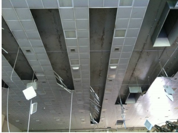
Fig. 2.24: Failure of a large suspended lightweight steel gypsum board ceiling, 2012 Emilia Earthquake, Mantova, Italy (photo courtesy by Marco Savoia)
