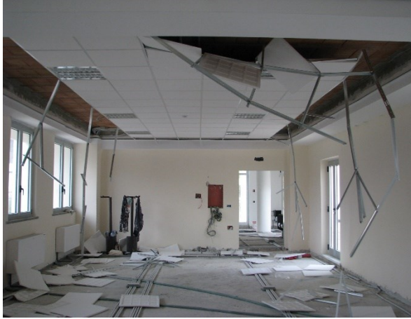
Fig. 2.26: Life safety risk: Damage to non-structural building components, 2009 Abruzzo Earthquake, L'Aquila, Italy (photo courtesy by Angelo Masi)
