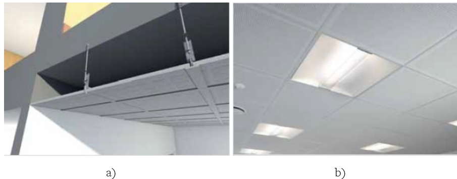
Fig. 2.12: Suspended acoustic lay-in tile ceilings: a) Integrated ceiling systems (photo courtesy by Knauf Italia); b) Example of a typical assembly (photo courtesy by Knauf Danoline)
