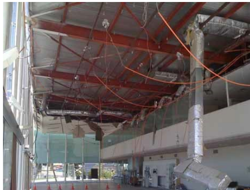
Fig. 2.20: Effects of the interaction between non-structural components and systems: Collapse of a suspended lightweight steel gypsum board ceilings due to the presence of a heavy HVAC ductwork in a commercial building, 2010 Chile Earthquake (photo courtesy by Knauf Chile)
