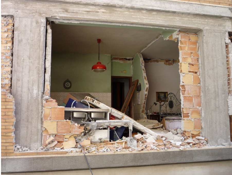
Fig. 2.1: Collapse of non-structural components in a residential building, 2009 Abruzzo Earthquake, L'Aquila, Italy
