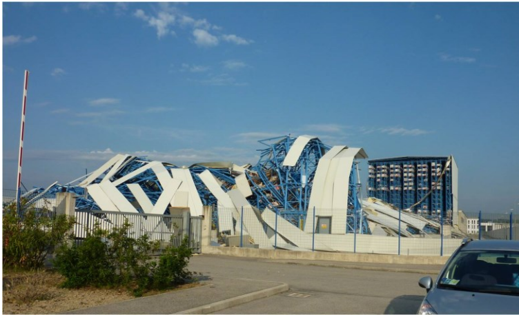
Fig. 2.27: Property loss risk: Damage to scaffolds in storehouses, 2012 Emilia Earthquake, Sant'Agostino, Italy (photo courtesy by Marco Savoia)
