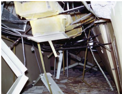
Fig. 2.29: Damage to non-structural components at the Olive View Medical Treatment Building, 1971 San Fernando Earthquake, Los Angeles, USA (photo courtesy by NISEE-PEER)
