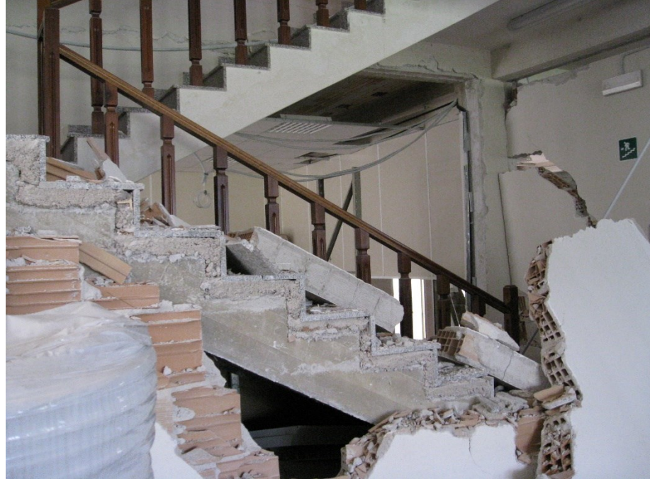
Fig. 2.2: Collapse of non-structural components in a storehouse, 2009 Abruzzo Earthquake, L'Aquila, Italy
