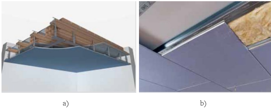
Fig. 2.10: Ceilings directly applied to the building structure: a) Example of a typical assembly (photo courtesy by Knauf Italia); b) Short-dropped furred gypsum board ceiling
