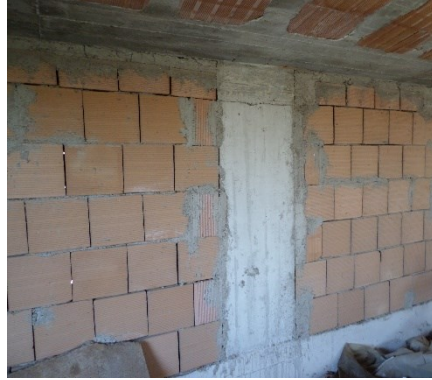
Fig. 2.8: Interior heavy partition wall
