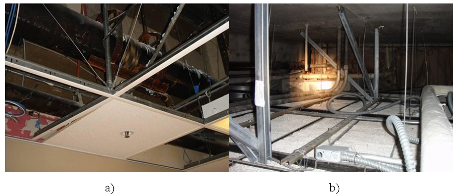
Fig. 2.34: Seismic bracings for suspended acoustic lay-in tile ceilings: a) Example of non-rigid bracing assemblies (FEMA, 2011); b) Example of rigid bracing assemblies (FEMA, 2011)
