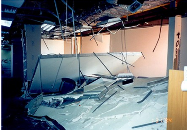
Fig. 2.22: Out-of-plane failure of an unbraced partial-height lightweight steel gypsum board partition wall due to the inertial forces, 1994 Northridge Earthquake, Los Angeles, USA (photo courtesy by Wiss, Janney, Elstner Associates, Inc.)
