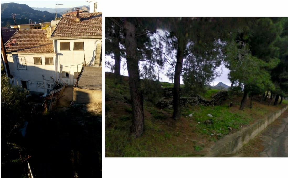
**Figure 6.95** Evidences of the landslides in Santa Severina: on the left, crack reported in a house within the redefined landslide in the NW sector; on the right, damaged retaining wall reported in the SW sector redefined landslides.
