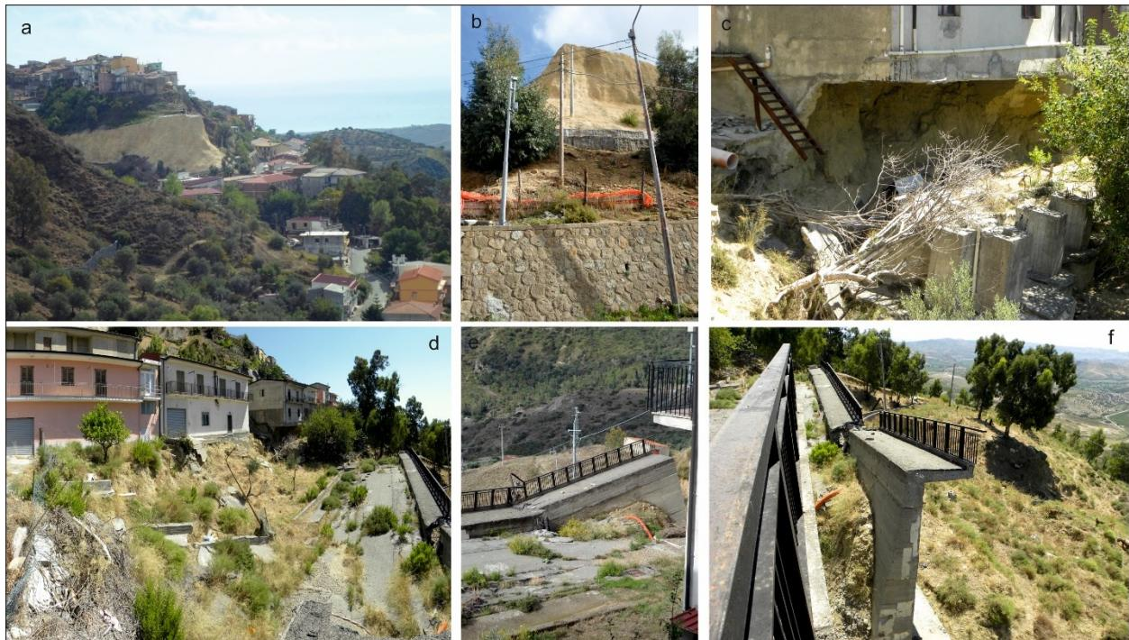
**Figure 6.8** a) View of the sandstone rock on which Cirò historical center is founded; b) particular of the rock, with also protective gabions; c) particular of the excavated foundation system of a house; d) damages on the road and on the houses in occurrence of the main scarp; e) view of Via de Gasperi from above; f) lateral view of Via de Gasperi (Photos taken during field survey, years 2013-2015).
