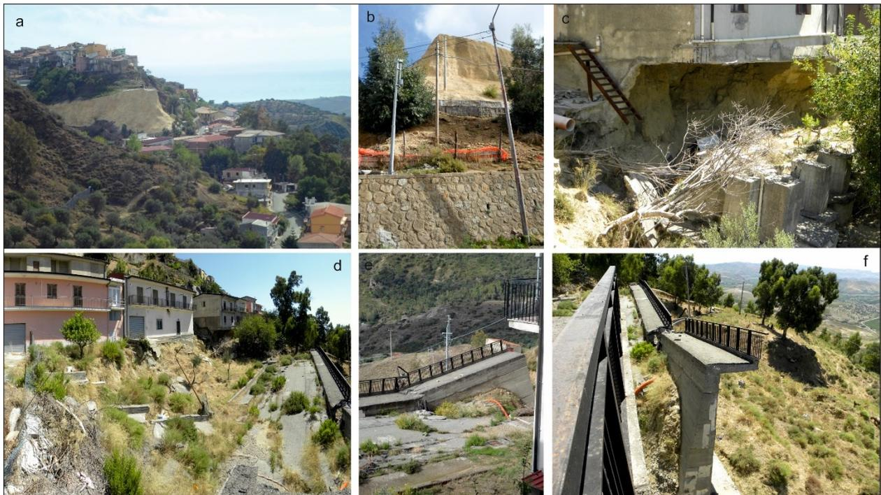
**Figure 6.8** a) View of the sandstone rock on which Cirò historical center is founded; b) particular of the rock, with also protective gabions; c) particular of the excavated foundation system of a house; d) damages on the road and on the houses in occurrence of the main scarp; e) view of Via de Gasperi from above; f) lateral view of Via de Gasperi (Photos taken during field survey, years 2013-2015).
