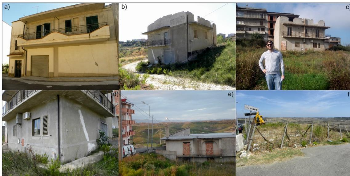
**Figure 6.25** Damage reported along the landslide main scarp and within the landslide body. a) fracture on a house located along the main scarp; b), c) and d) damage reported on an abandoned house inside the Southern landslide; e) damage reported on an abandoned house inside the Northern landslide; f) fences and road signs clined downwards.
