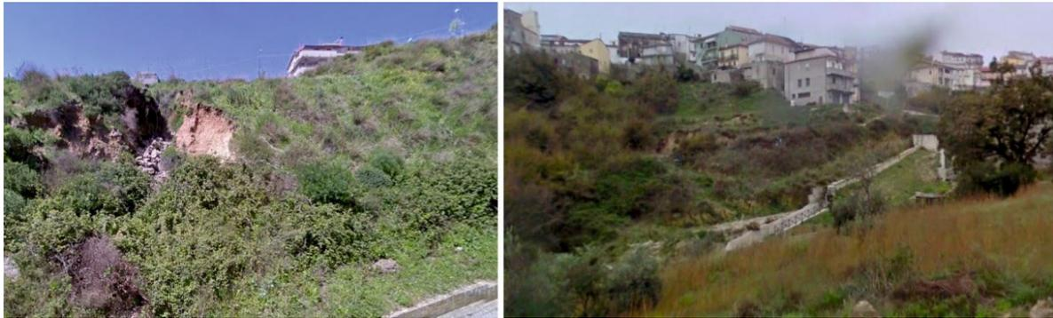
**Figure 6.104** Evidences of the landslides in Scandale: on the left, evidences of the new landslide in the SW sector; on the right, fracture in the new landslide in the SE sector.
