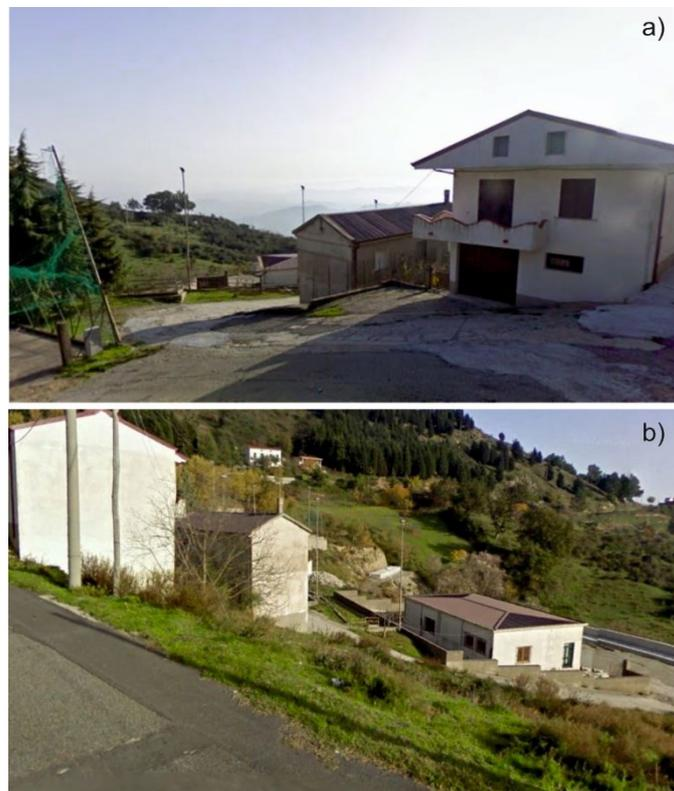
**Figure 6.74** Evidences of the SE landslide in S. Nicola dell'Alto. a) tilted electric lights and damage on the house; b) on the background, evidences of loose soils.
