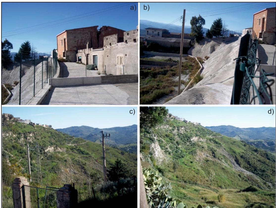
**Figure 6.59** Evidences of the redefined landslide in the South-facing slope of Crucoli.a) and b) damage reported on an abandoned house and remedial works on the slope. c) and d) Flow-type landslide reported in the southern part of Crucoli.
