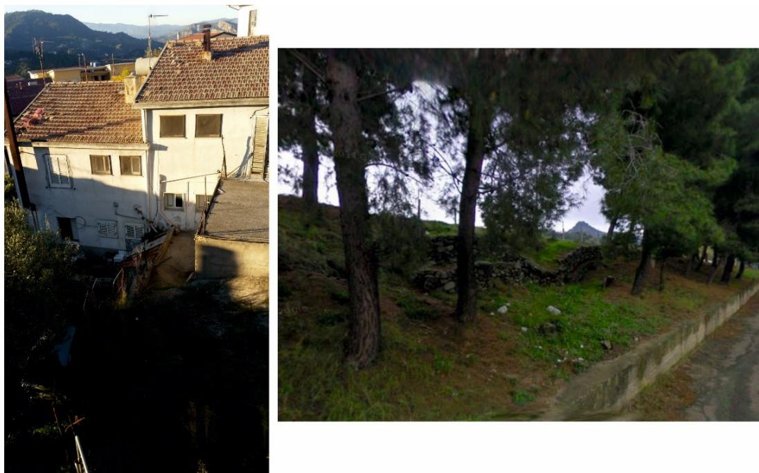
**Figure 6.95** Evidences of the landslides in Santa Severina: on the left, crack reported in a house within the redefined landslide in the NW sector; on the right, damaged retaining wall reported in the SW sector redefined landslides.
