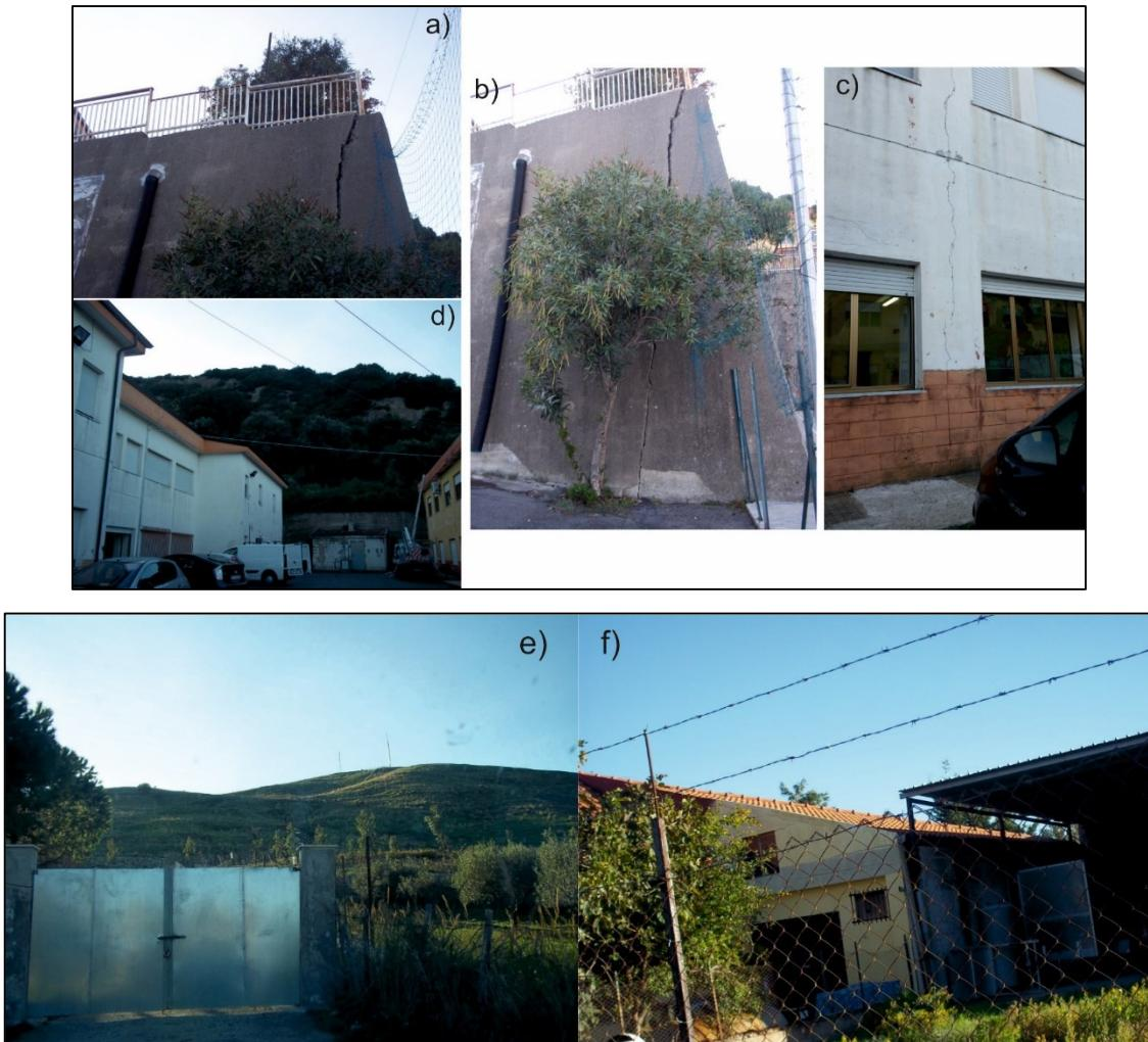
**Figure 6.69** Evidences of the northern landslide in Melissa, on the top, and of the continuous landslide in Torre Melissa, on the bottom. a) and b) fracture in a retaining wall; c) fracture in the school, d) oblique view of the school and of the rocky slope in the background; e) concavity-convexity landscape in Torre Melissa; f) fractures reported in a house in Torre Melissa).
