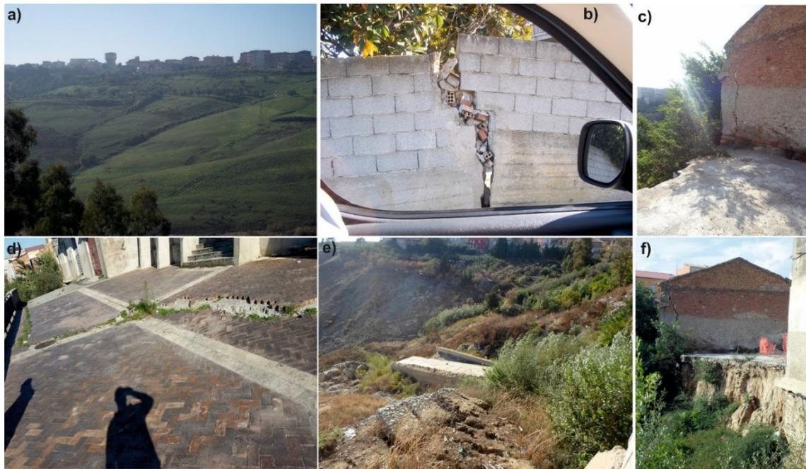
**Figure 6.109** Evidences of the landslides in Cutro: a), concavity and convexity of the redefined landslide in the Northern sector b) crack in a wall within the redefined landslide in the Northern sector; c), d), e), f) damage to house, to roads and to remedial works within the redefined landslide in the Southern sector.
