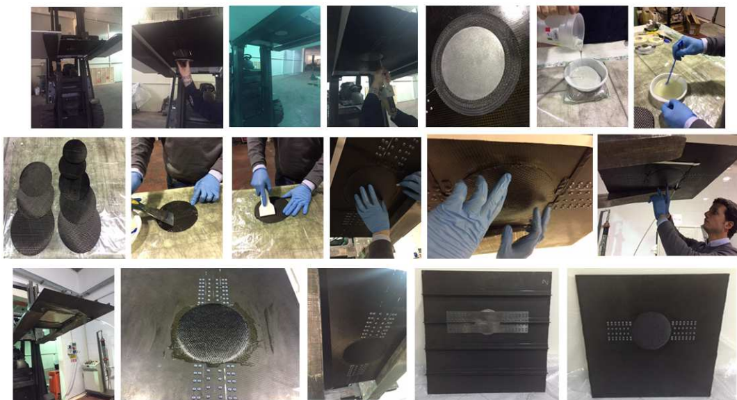
Figure 102 - Implementation of the AER Project repair (2)
