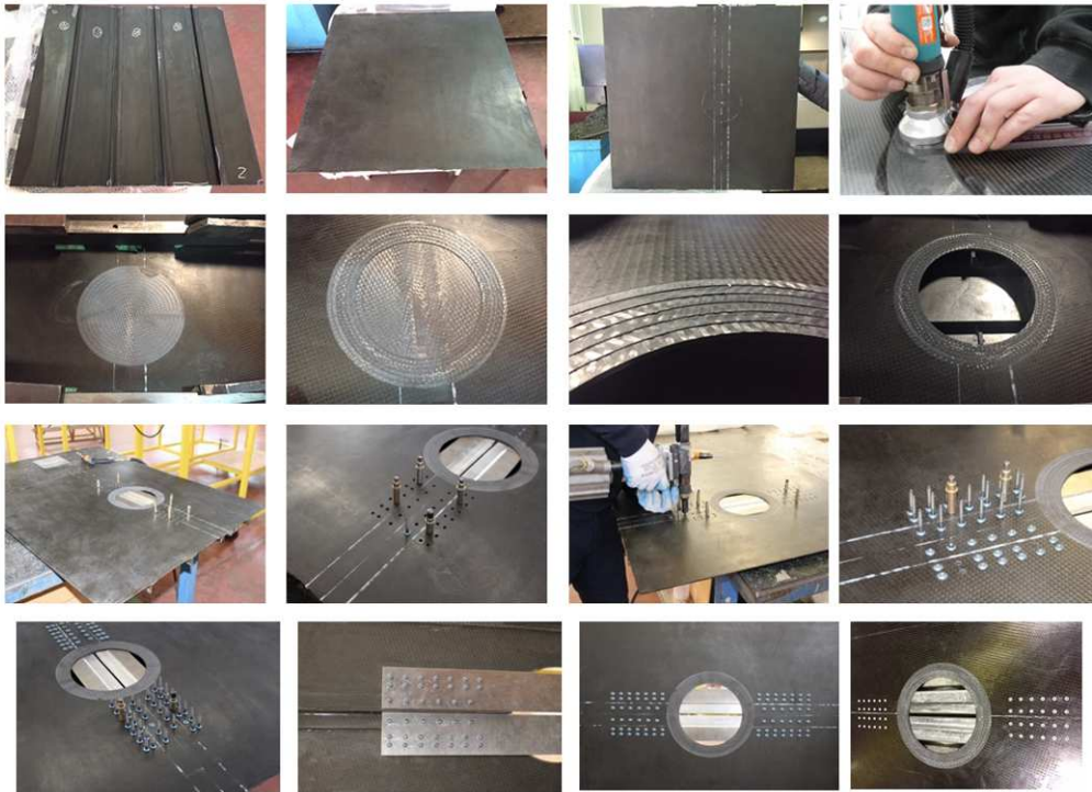
Figure 101 - Implementation of the AER Project repair (1)
