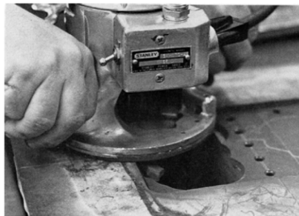
Figure 23 - Damage Removal with Hand Held Router
