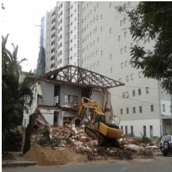
Figure 4.17 – Old colonial house demolished to create space for a new tall-building
