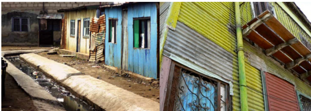
Figure 4.58 – Houses in zinc and wood in Mafalala
