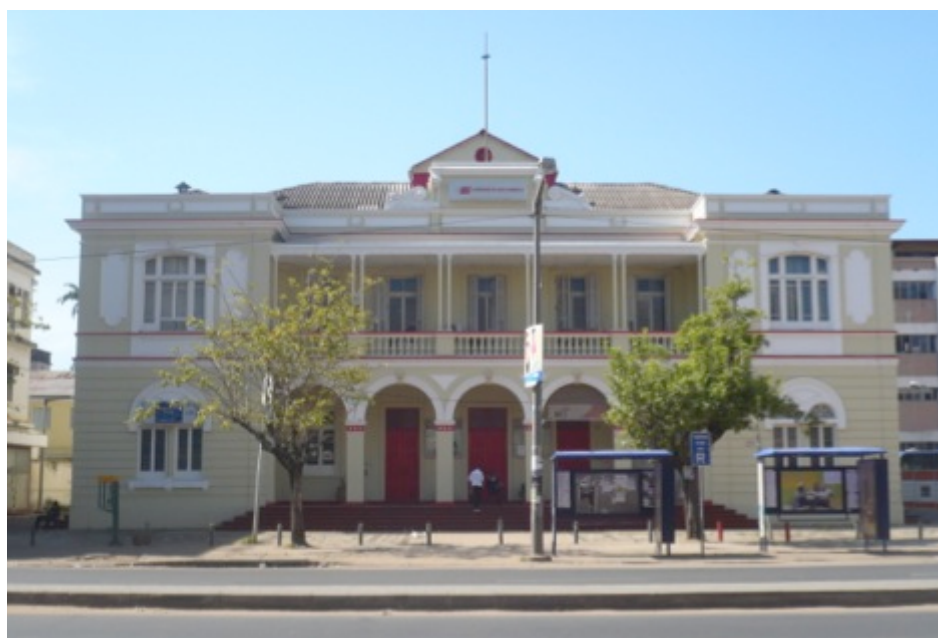
Figure 4.30 – Maputo Post Office Building
