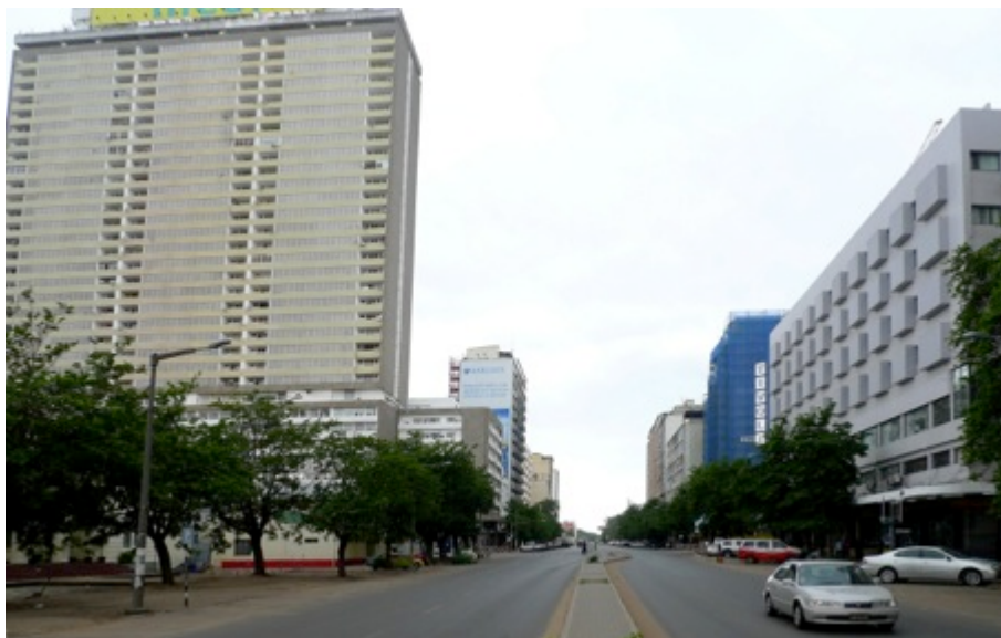
Figure 5.17 – The Thirty-three Floors Building
