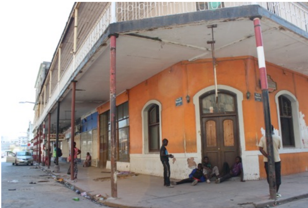
Figure 4.18 – Colonnaded building downtown (Baixa) in a state of degrade
