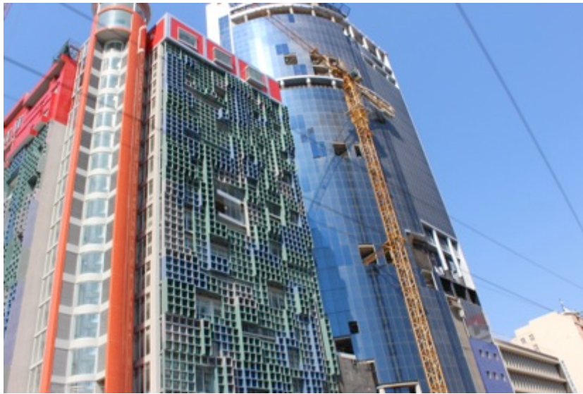
Figure 4.7 – New premises of Bank of Mozambique in the Baixa
