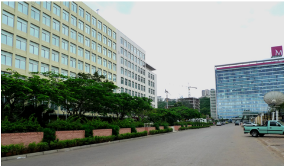
Figure 5.21 – Location of the area of new construction under the green zone of protection
