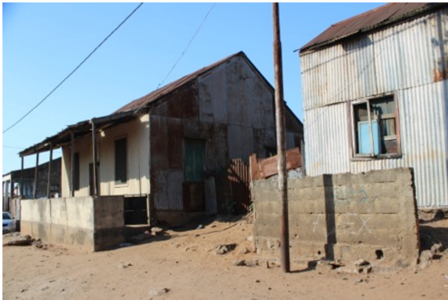
Figure 4.56 – Typical house in zinc and wood in Mafalala informal settlement
