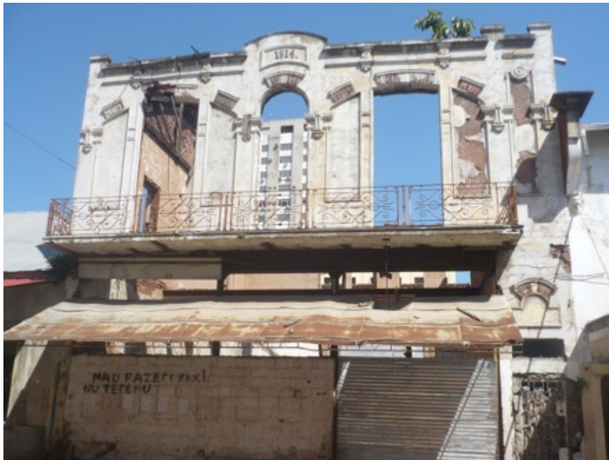
Figure 4.15 – Also many structures built before 1920 are abandoned and deteriorated
