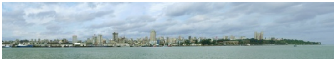
Figure 5.1 – Skyline photo of the area of intervention
