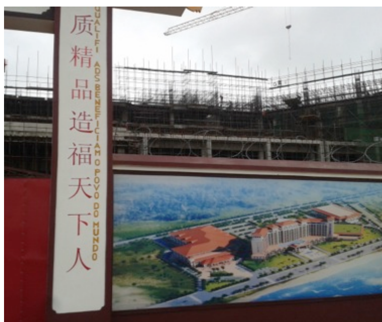
Figure 4.6 – Construction of a five stars resort along Avenida Marginal
