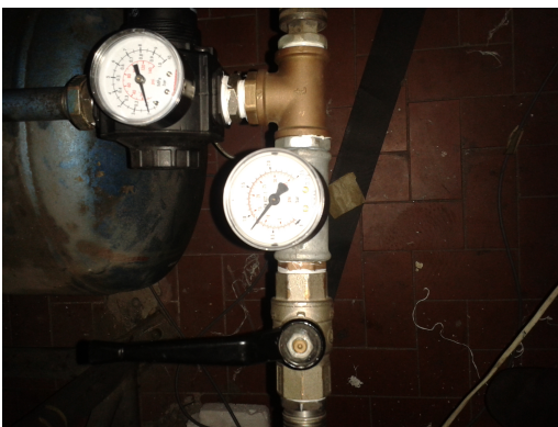
(b) Main tank pressure control unit
