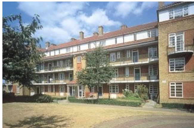
Acorn Walk, Surrey Docks, before and after refurbishment (fonte http://www.lddc-history.org.uk/ )
