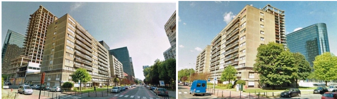
Brussels, Belgium, Chausée d'Anvers 61-63 (fonte Studio Samyn, Brussels)
