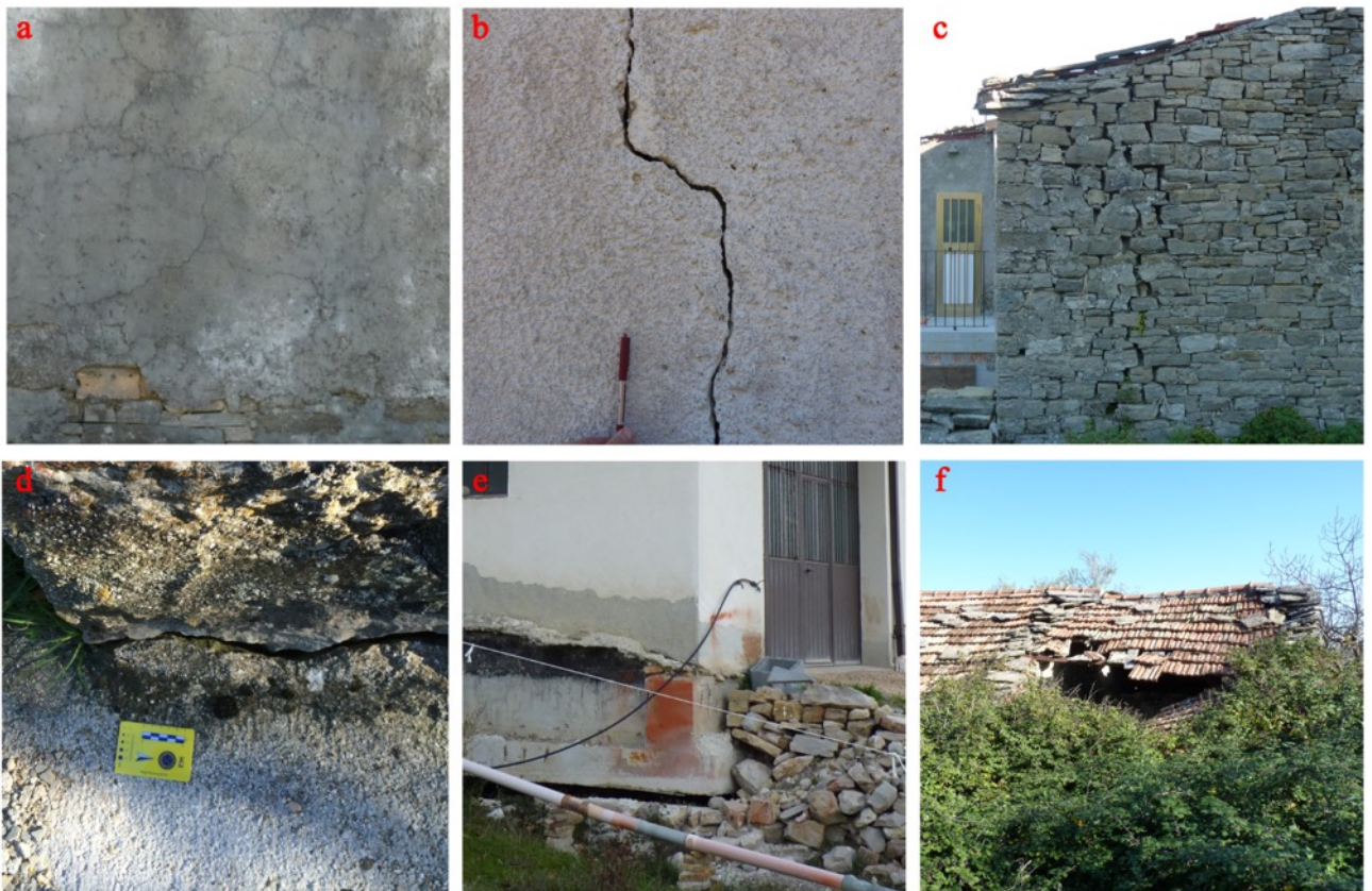
Fig. 5.26 - Example of cracks and rupture identified on structures. a) hairline cracks on plaster of masonry wall; b) open crack on reinforced concrete walls; c) open crack of masonry building walls; d) open crack between wall and external sidewalk; e) open crack between external wall and ground surface; f) collapsed roof in a masonry building (Del Soldato et al., under review_a)
