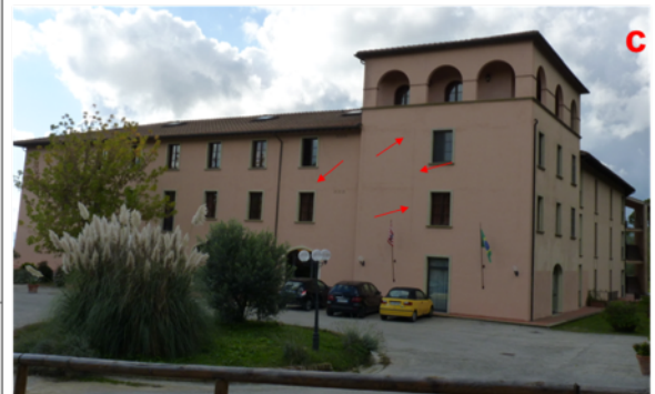
Fig. 5.63 - Sample of the recording scheme (Del Soldato et al., under review_b) compiled (a), with two images (b and c) of the investigated buildings, used for the recognition of the damage affecting the several surveyed structures in the southwestern sector of Volterra.
