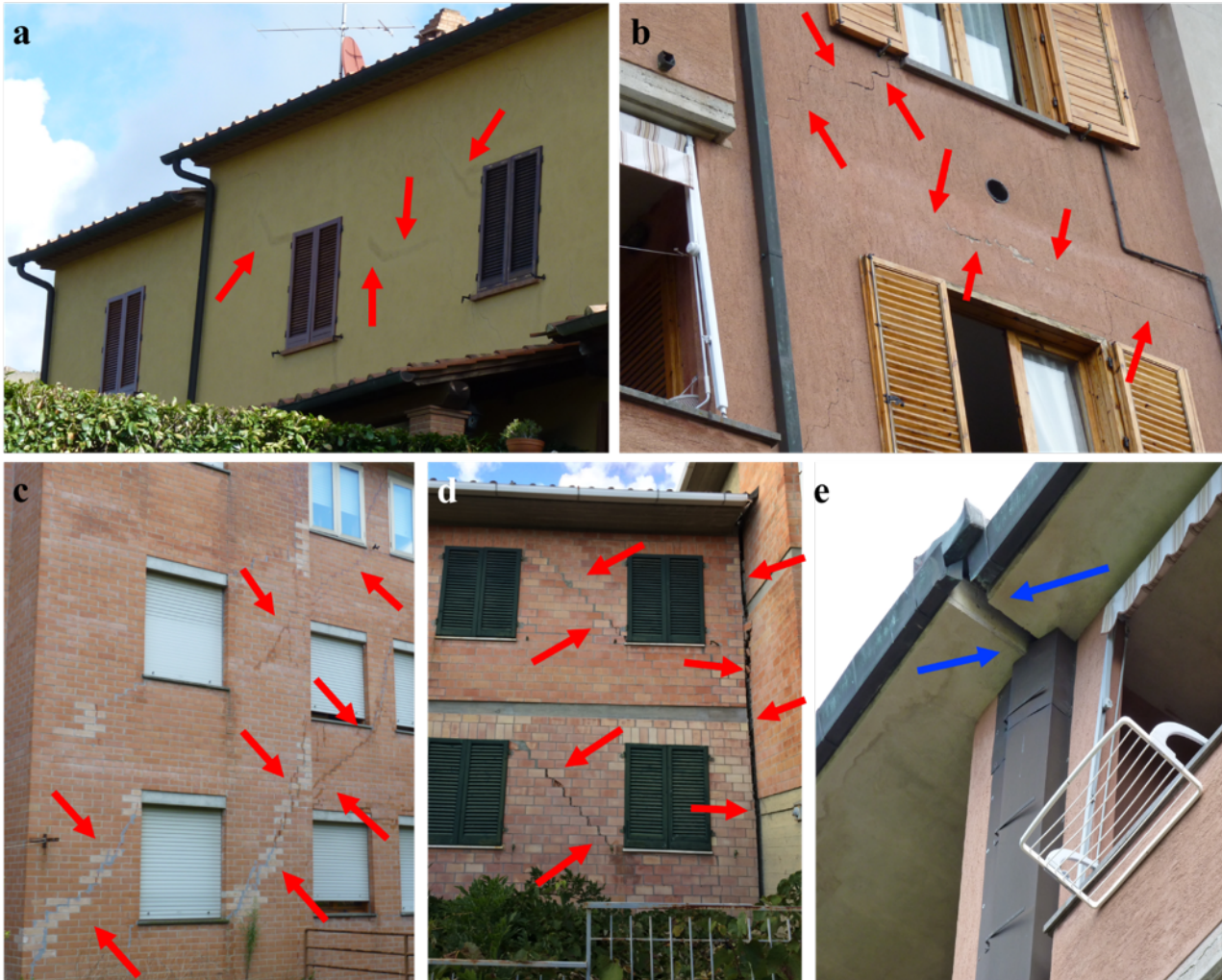
Fig. 5.62 - Different types of damage (red and blue arrows) recognized during field surveys on buildings in the southwestern sector of Volterra. a) plaster cracks restored; b) weak and moderate fractures on plaster; c) numerous severe fractures; d) important cracks plunging about 45° and open fractures between the two structures; e) important tilting between two parts of the same buildings.
