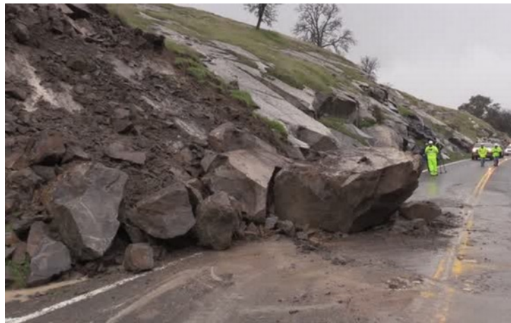
Fig. 2.8 - Rock slide occurred on the Highway 41 in Madera County on, Jan. 19, 2016 ( http://www.fresnobee.com/news/local/article55419970.html ).
