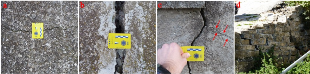
Fig. 5.27 - Fine (a) and open (b) cracks recognizable on pavement of sidewalks slab; hairline (highlighted by means of red arrows) and open fractures on concrete (c) and masonry walls (d).
