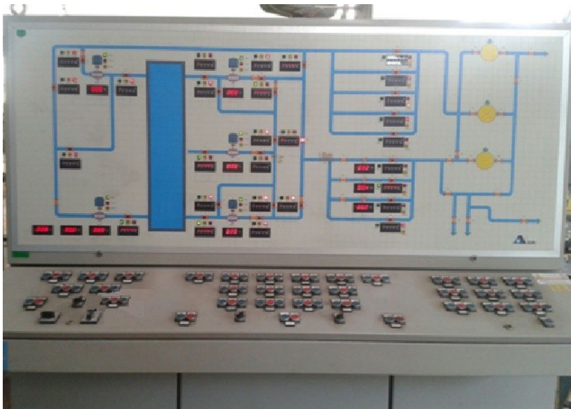
Fig. 4.5 Control panel of the pump station
