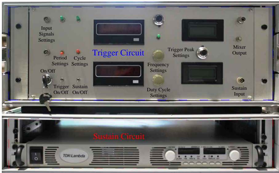
Figure 6.4: Front view of the power supply system. The top box contains the trigger circuit, the bottom one includes the sustain circuit.
