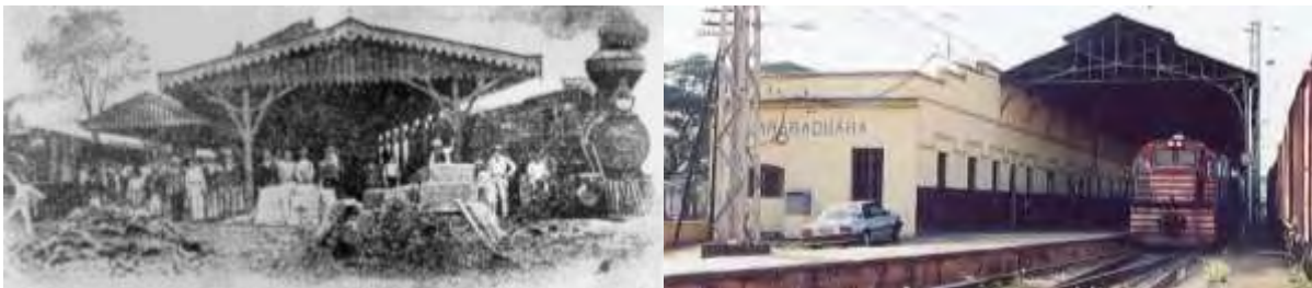
Fig. 10 Araraquara railway station in 1910 and 2002. Fonte: W. L. C. Barcellone (2009)
