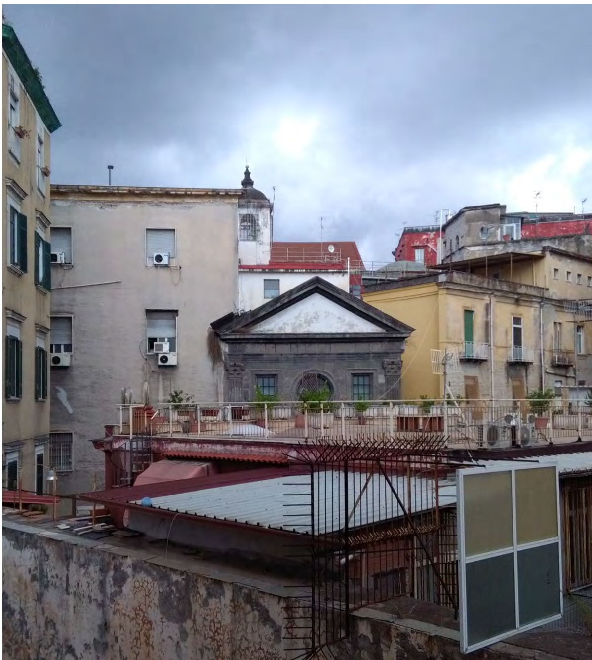
St. Mary Mater Domini: View from the roofs
