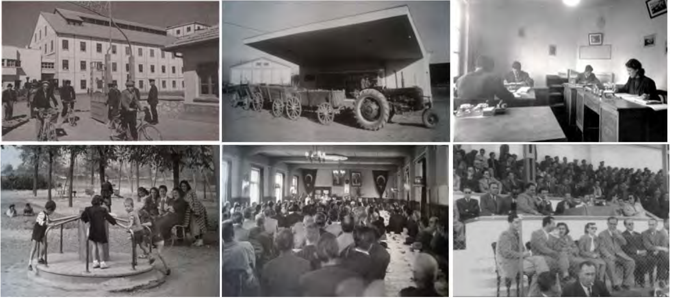
4: Daily routines and social practices in Eskişehir Sugar Factory (Eskişehir Sugar Factory archive).
