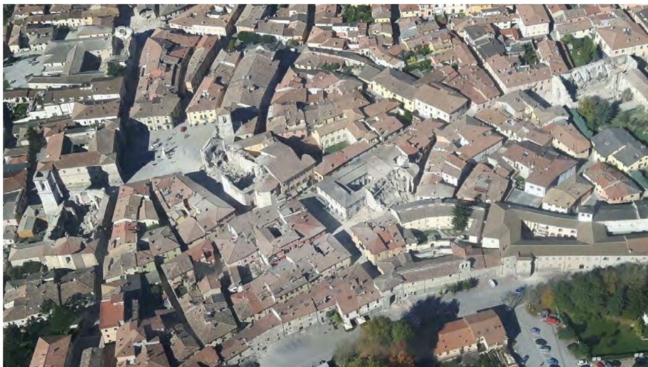
2: Norcia (Perugia). Damage caused by the 2016 earthquake.
