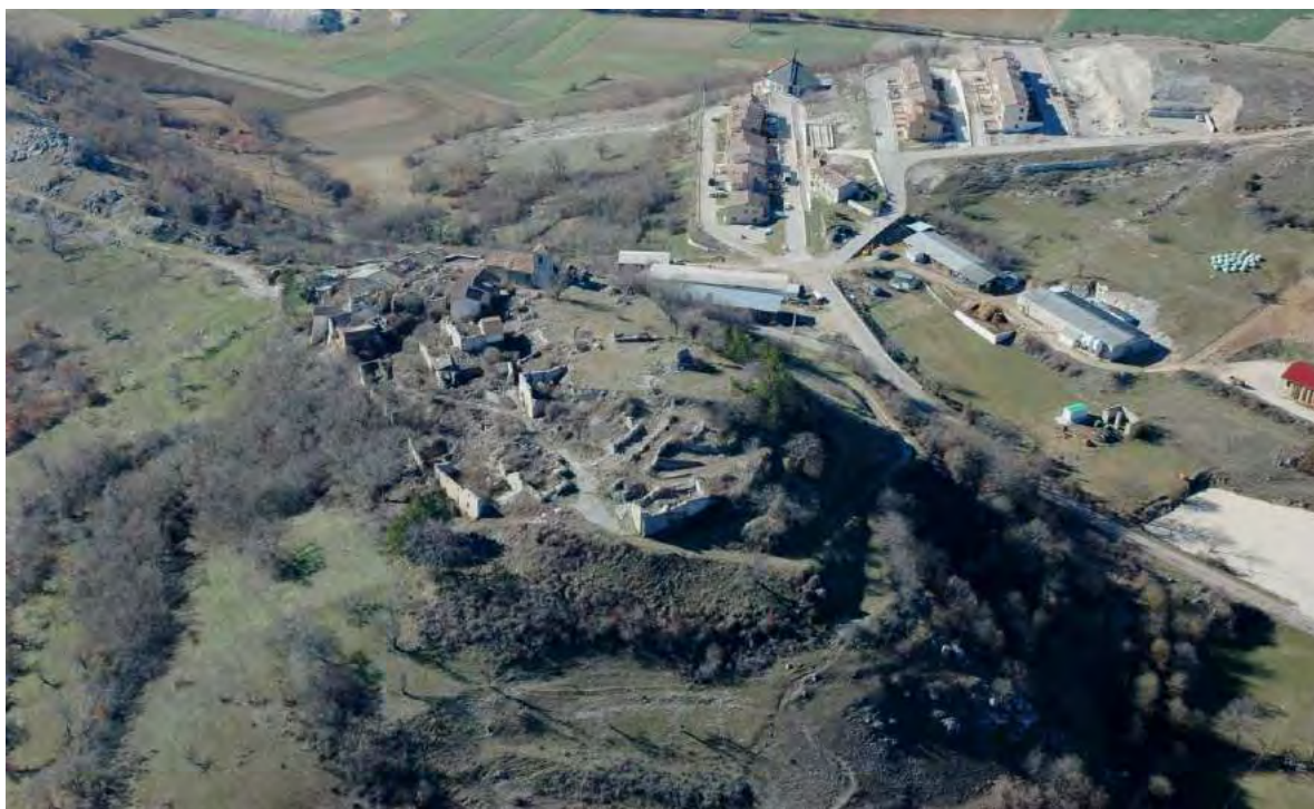
4: Chiavano (Cascia, Perugia). The translated reconstruction of the historical center after the 1979 earthquake.
