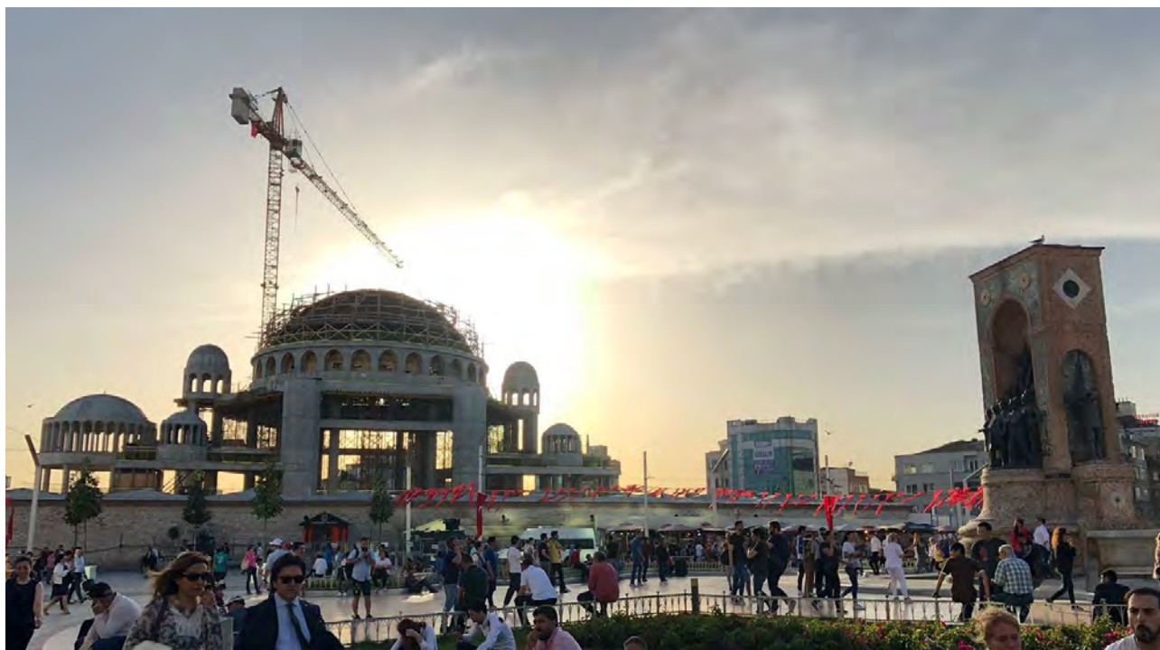
4: Republican Monument and the construction of Taksim Mosque at Taksim Square [photographed by the author, 18.05.2018].
