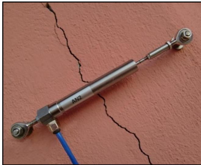
Figure 6.20 Example of crack-meter to monitoring movement of crack.
