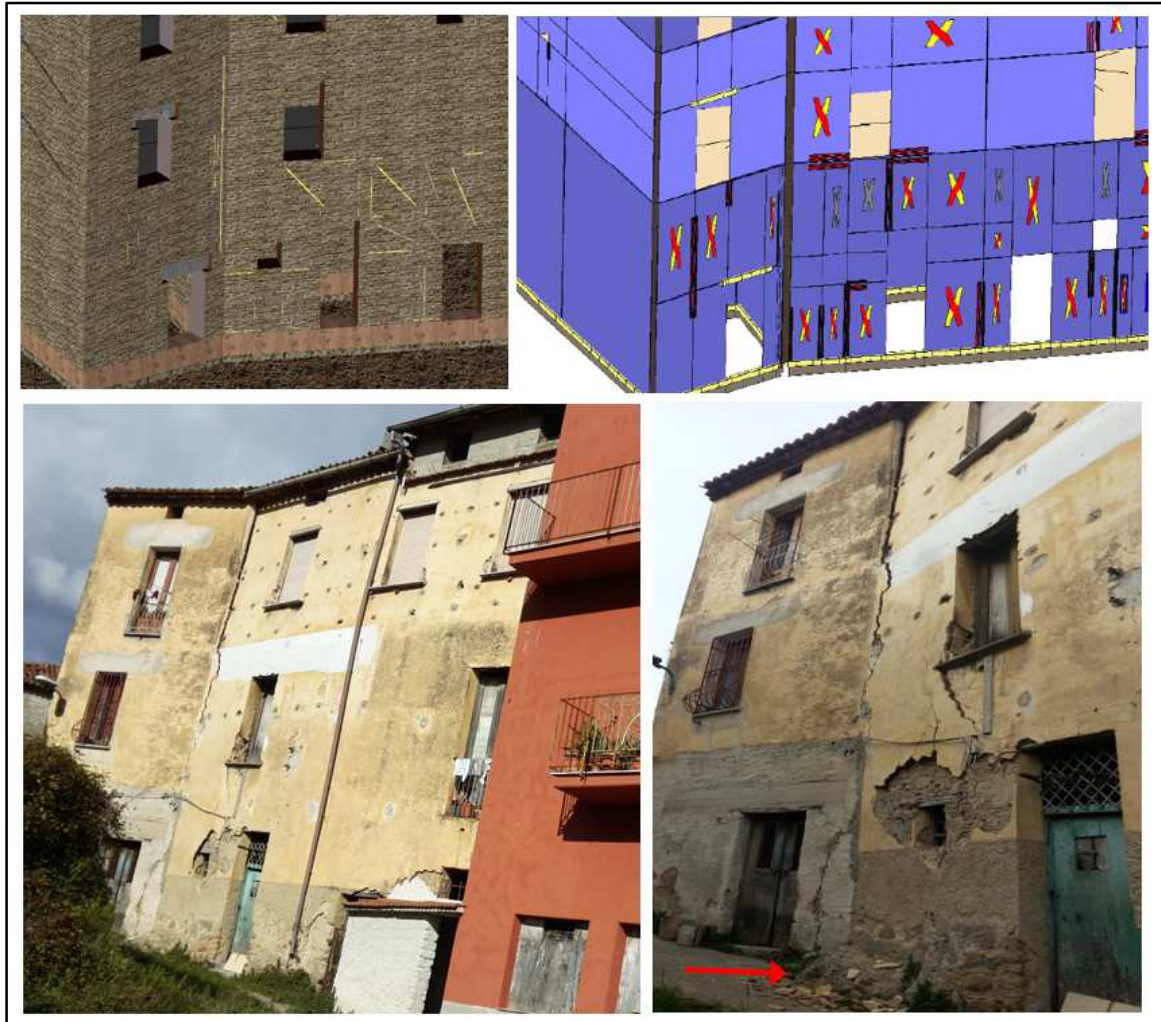
Figure 8.158 Comparison between damage distribution obtained by computational model (on the top) and surveyed by in situ campaign in February 2015 (on the bottom) on building façade more damaged.
