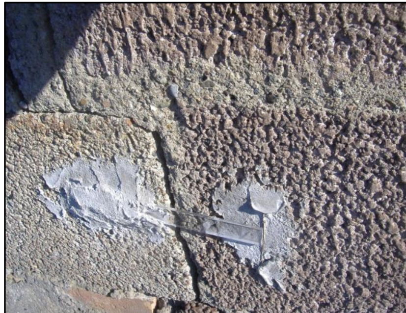
Figure 6.18 Glass crack monitoring system.
