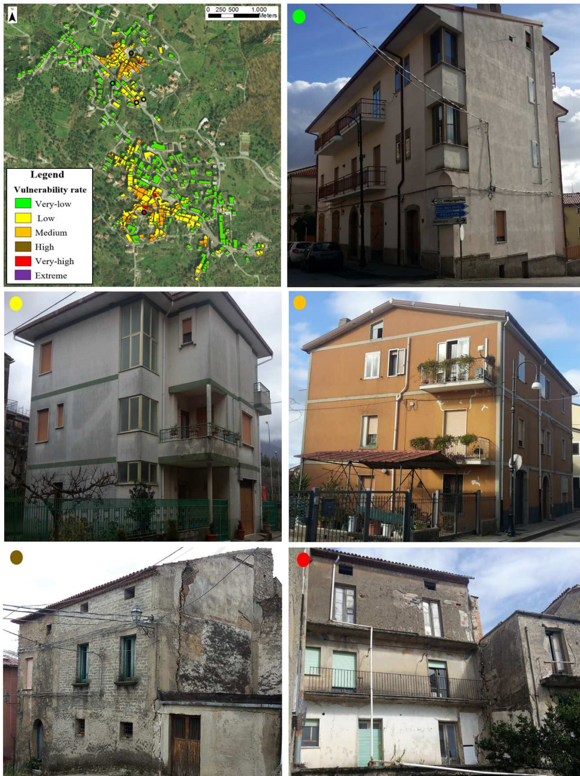
Figure 8.82 Buildings with different vulnerability level in Moio della Civitella urban center.
