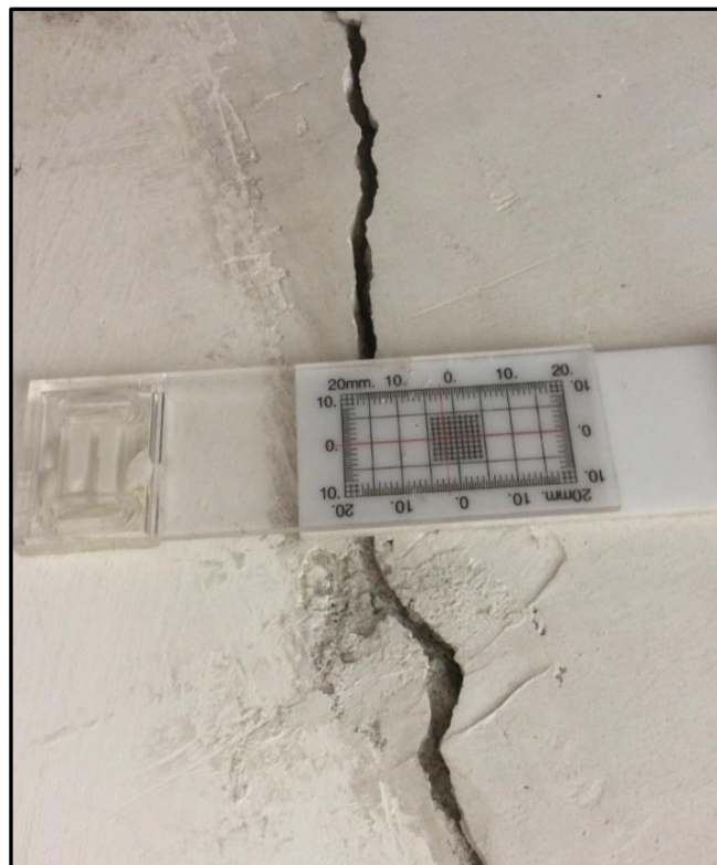
Figure 6.19 Example of “Tell Tale” crack monitoring.
