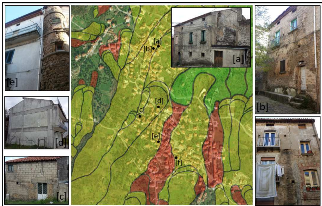
Figure 8.60 Examples of damage occurred to buildings within dormant landslide affected areas.
