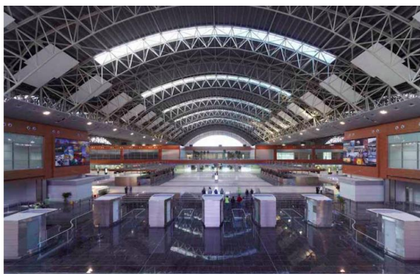
Figure 1.5 Sabiha Gökçen International Airport, Istanbul Turkey (Image Source: Arup)
