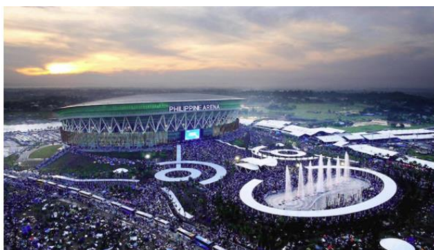
Figure 1.10 Philippine Arena (Image Source: Philippine Arena)
