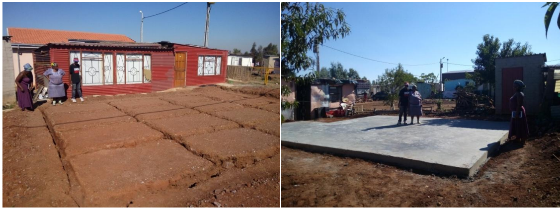
Fig.5.7 | Foundations of the future houses of the Fedup scheme
