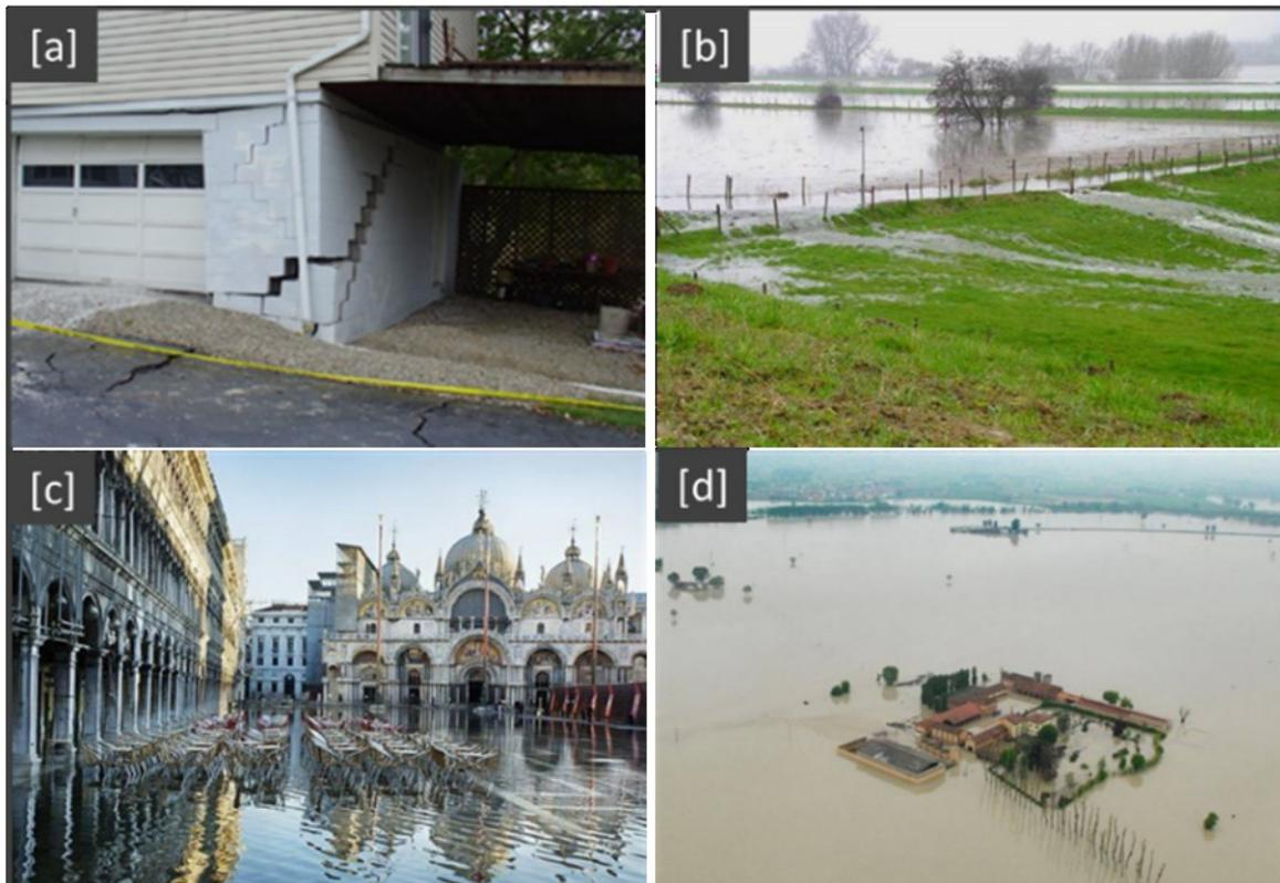
**Figure 1.1** – Examples of effects associated to subsidence: (a) house cracking in America; (b) change in surface water drainage in Holland; (c) landward incursion of seawater in Venice, Italy; (d) flooding in Italy.
