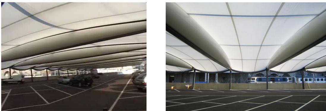
Figure 1.6: Tensairity Structure; Garage di Montreux Station, Montreux (Swiss), R. Luscher.
