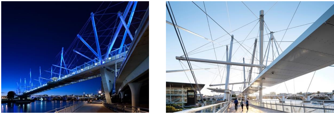
Figure 1.5: Tensegrity Structure; Kurilpa Bridge, Queensland (Australia), Ove Arup & Partners.
