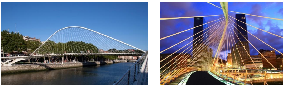
Figure 1.3: Cable structure; Zubizuri Bridge, Bilbao (Spain), S. Calatrava.
