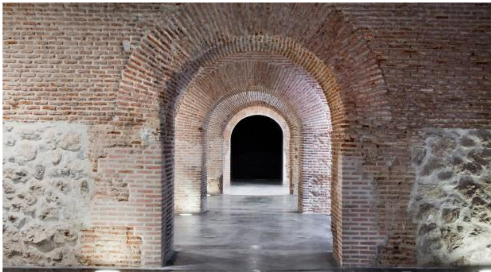
Fig. 3.14 – Detail in the zone of bovedas .
