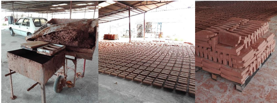
Fig. 4.1 - Brick construction and air-drying phases
