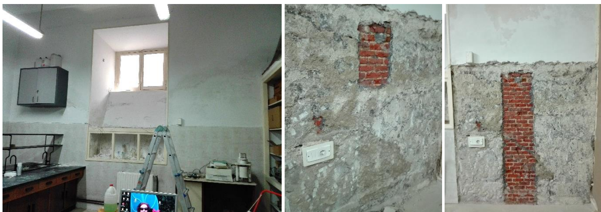
Fig. 6.10 – The wall before and after the removal of the plaster
