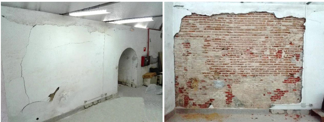
Fig. 6.3 – The wall before and after the removal of the plaster
