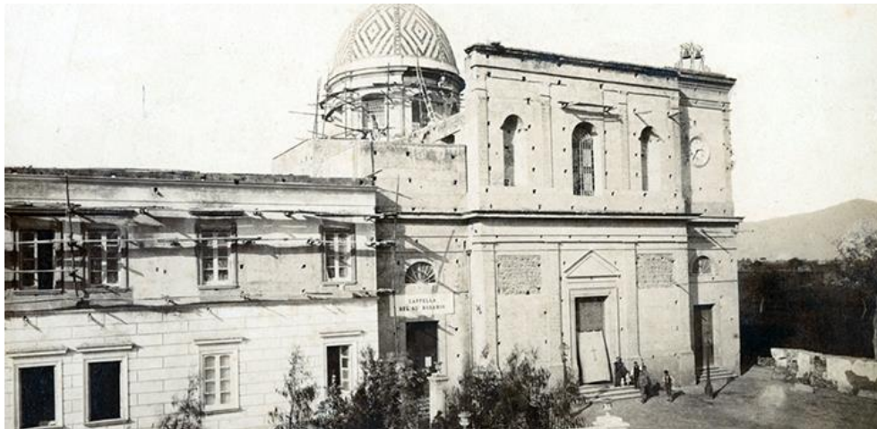
Fig. 3.25 – The Sanctuary before the enlargement and works on the facade.
