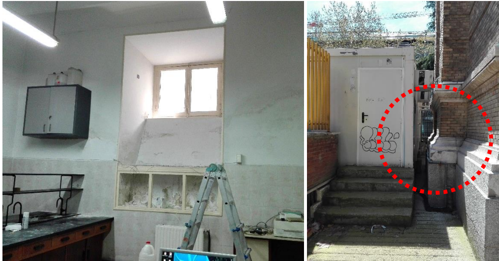
Fig. 3.24 – Identification of the area of intervention
