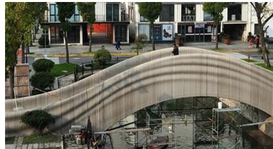
Figure 1.2. First 3D-printed bridge realized in Shanghai
