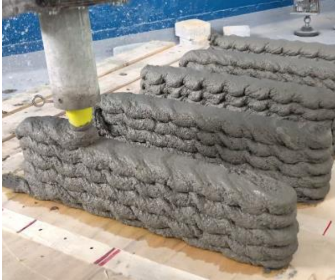
Figure 3.9. Printing of concrete elements
