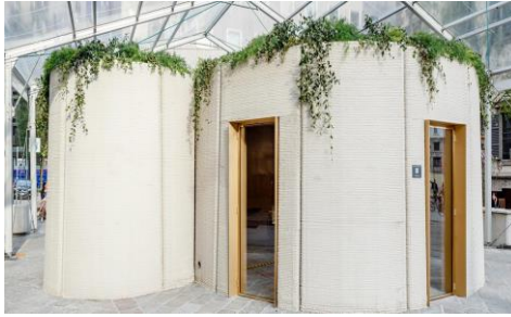
Figure 1.1. First 3D-printed house produced in Italy
