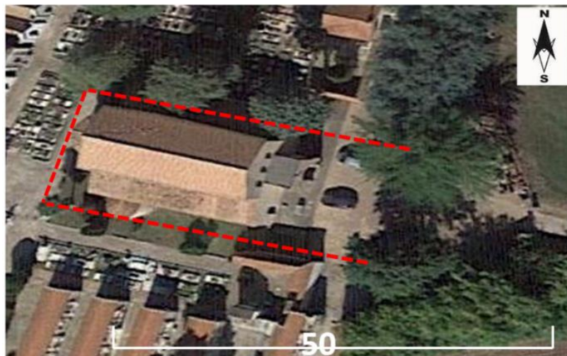
Figure 2.22 U-shaped electrode distribution along three external perimeter walls (dashed red lines) of the Basilica of Santa Maria near Alvignano village (northern Campania Region, southern Italy) (modified from Bottari et al., 2020).
