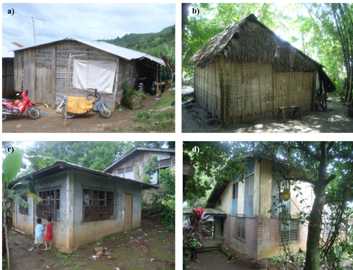
Fig. 7.3 a) typical nipa hut with thatched roof, b) typical timber frame dwelling with metal sheet roof, c) typical reinforced concrete frame building with metal sheet roof, d) typical mixed construction building with a lower reinforced concrete frame and upper timber frame with timber boards. (Jenkins et al., 2014)
