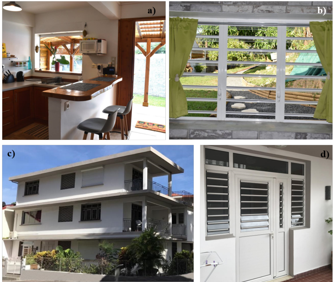
Fig. 7.14 a) example of absence of window's frame, b) typical UPVC louvre shutters, c) Example of uPVC roller shutters in new buildings, d) typical mixed UPVC windows and doors frame. (Google Earth Pro)
