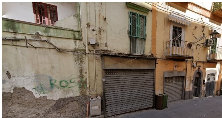
Fig. 6.39 Examples of steel shutters in the municipality of Torre del Greco (Google Earth Pro)
