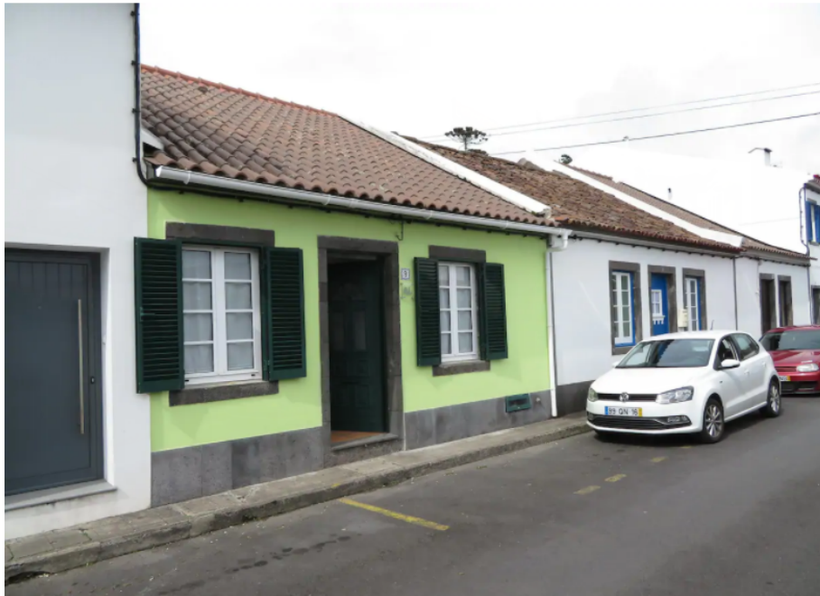
Fig. 7.10 Example of UPVC louvre shutters in the analysed area of Furnas (Google Earth Pro)
