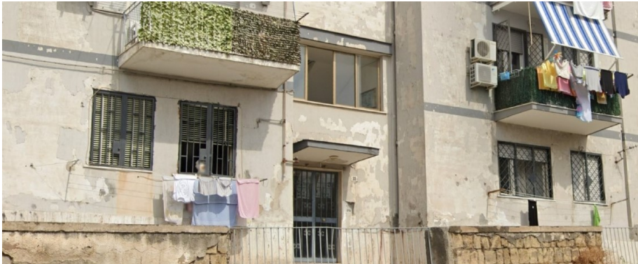
Fig. 6.43 Examples of steel shutters in the municipality of Ercolano (Google Earth Pro)
