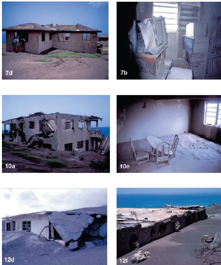
Fig. 3.13 Soufrière Hills volcano eruption, Montserrat, December 1997. Damage produced by a pyroclastic flow: a) in a peripheral zone of the flow; b) in an intermediate zone of the flow; c) in the central zone of the flow. (Baxter et al., 2005) [2]
