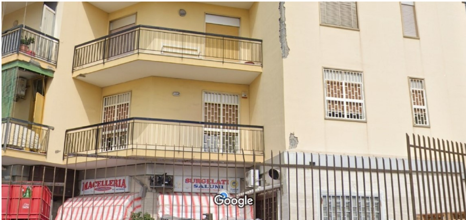
Fig. 6.42 Examples of steel shutters in the municipality of Ercolano (Google Earth Pro)
