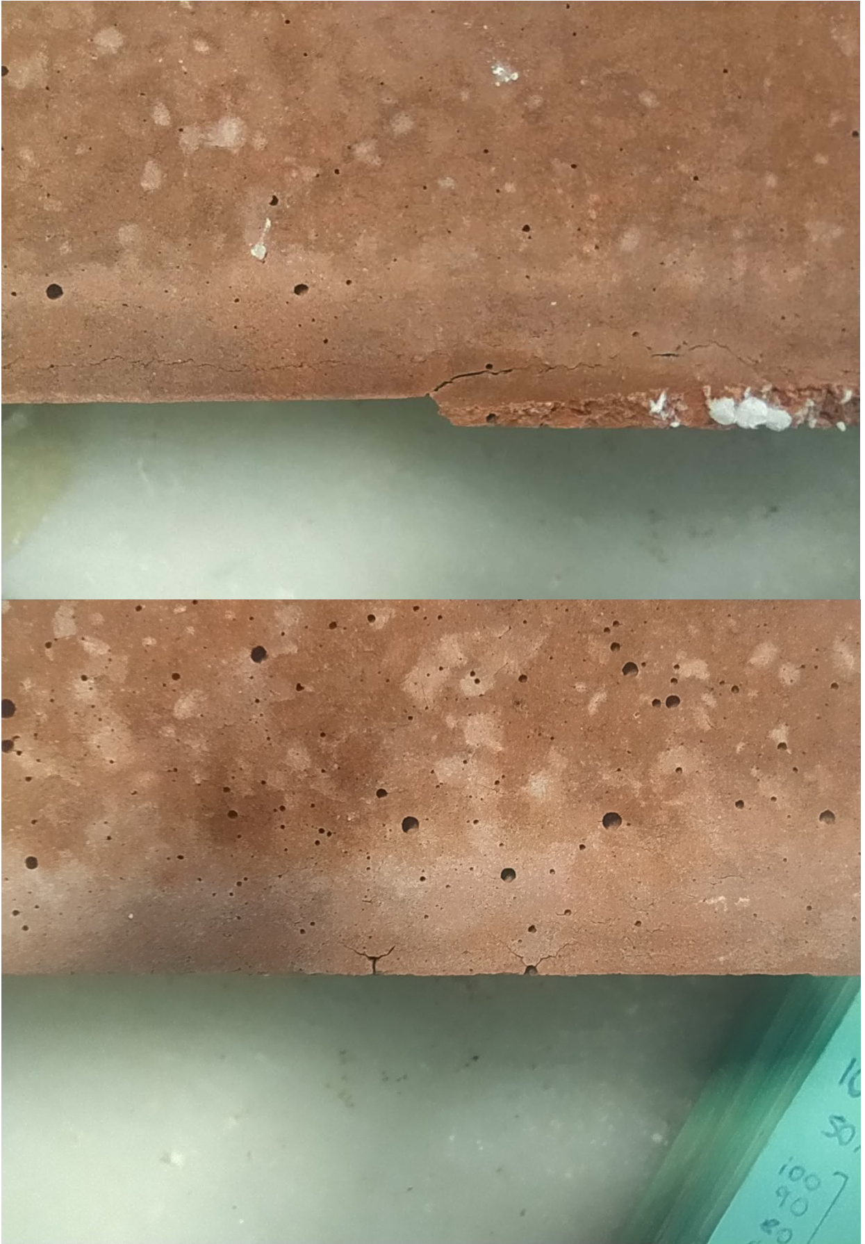
Figure 136 - Matting, cracking and efflorescence
