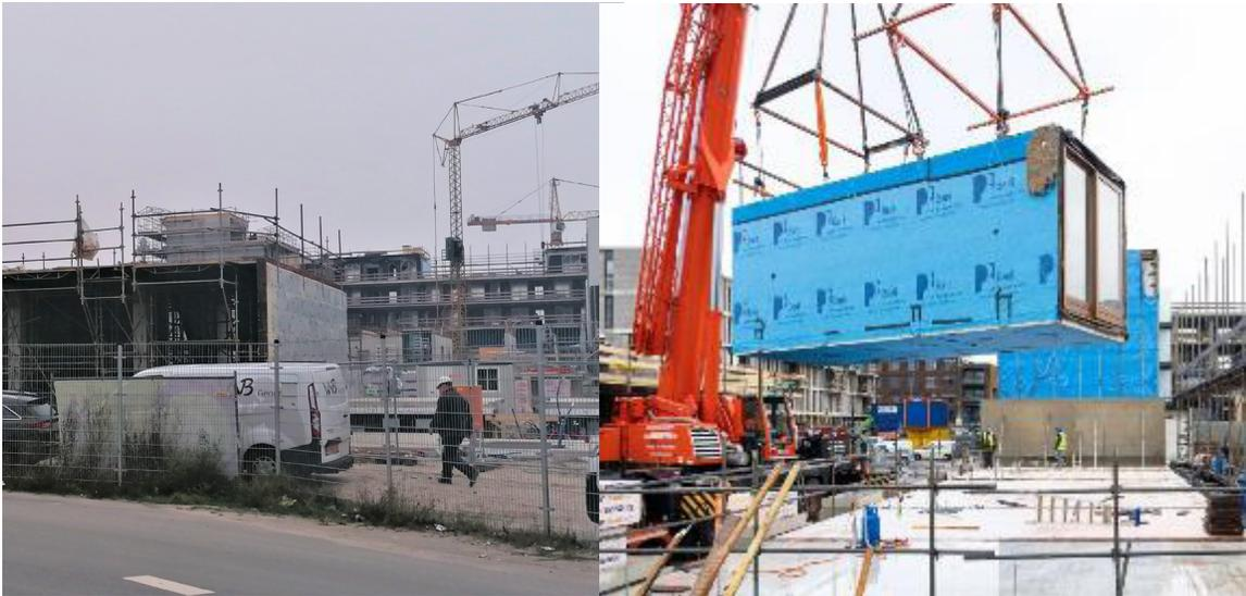
Figura 43. The construction technique with prefabricated modules responds to the need for adaptability of space (reducing demolition waste) and prevents from new construction waste on site. Source: left: (Search, 2018b)- Righ: author's photo 2021.
