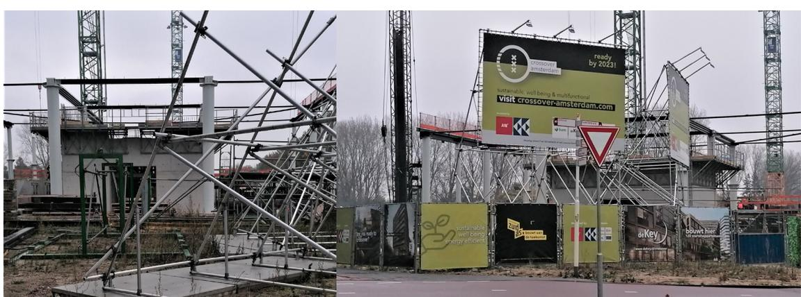
Figura 38. To reduce the production of waste (on the construction site and in the demolition phase), cement is used only for the construction of the stairwell and elevator shaft. Photographs of the author 2021.
