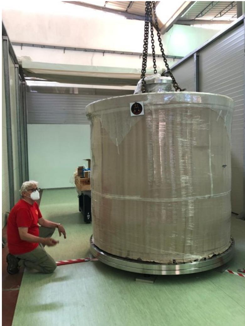
Figure 4.7: Installation of the cryostat in the Planck Hall
