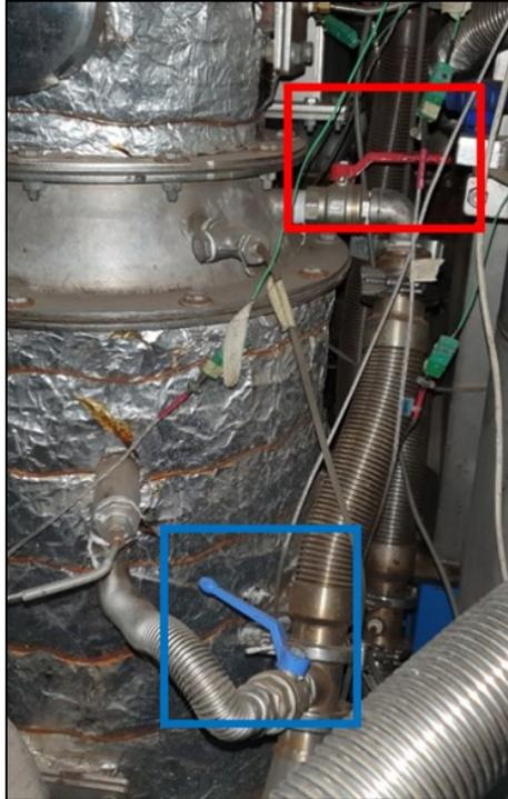
Figure 3. 8: Installation of ball valves on CMD ECO20x.
