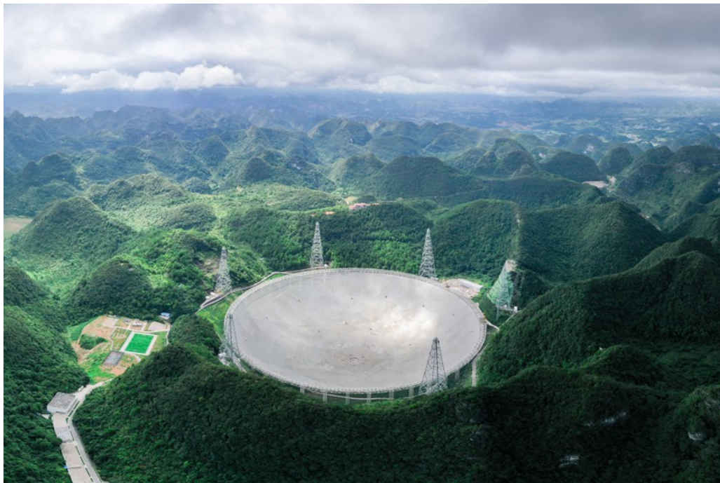
Figure 2.1. A spectacular bird-view of the FAST Radio Telescope in Pingtang county, China. The telescope observes the radio sky between 70 MHz and 4 GHz with an angular resolution of 4 arcseconds.
