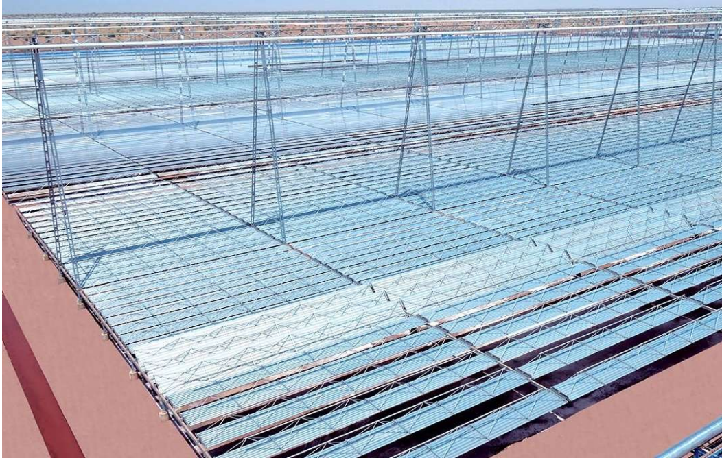
Figure I.3 A linear Fresnel reflector in Dhursar village in Rajasthan, India (Dhursar CSP, 125 MW).
