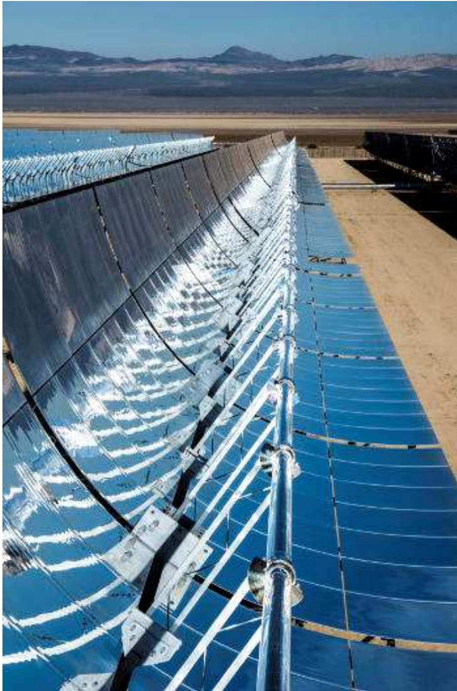
Figure I.2 A parabolic trough in the Mojave Desert in California, USA (Mojave Solar Project, 250 MW).
