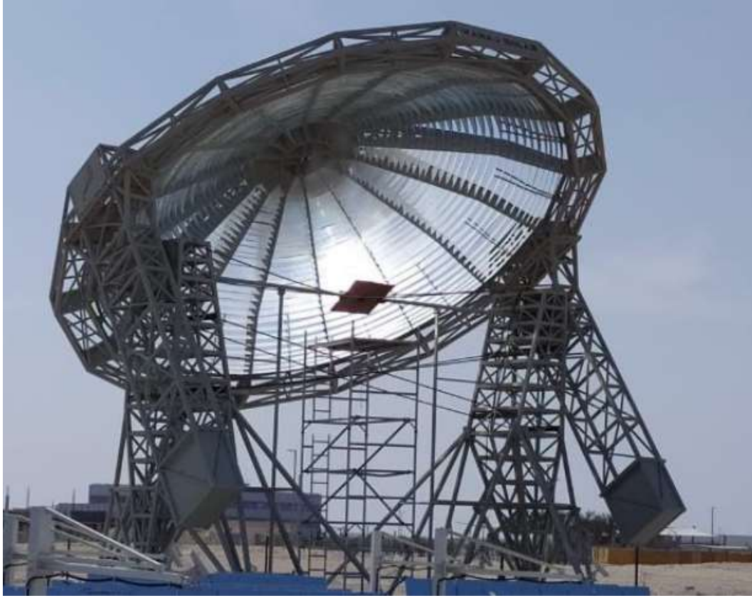
Figure I.7 The spot Fresnel reflector at the Masdar Institute Solar Platform near Abu Dhabi, United Arab Emirates (ASC-10, 10 kW).
