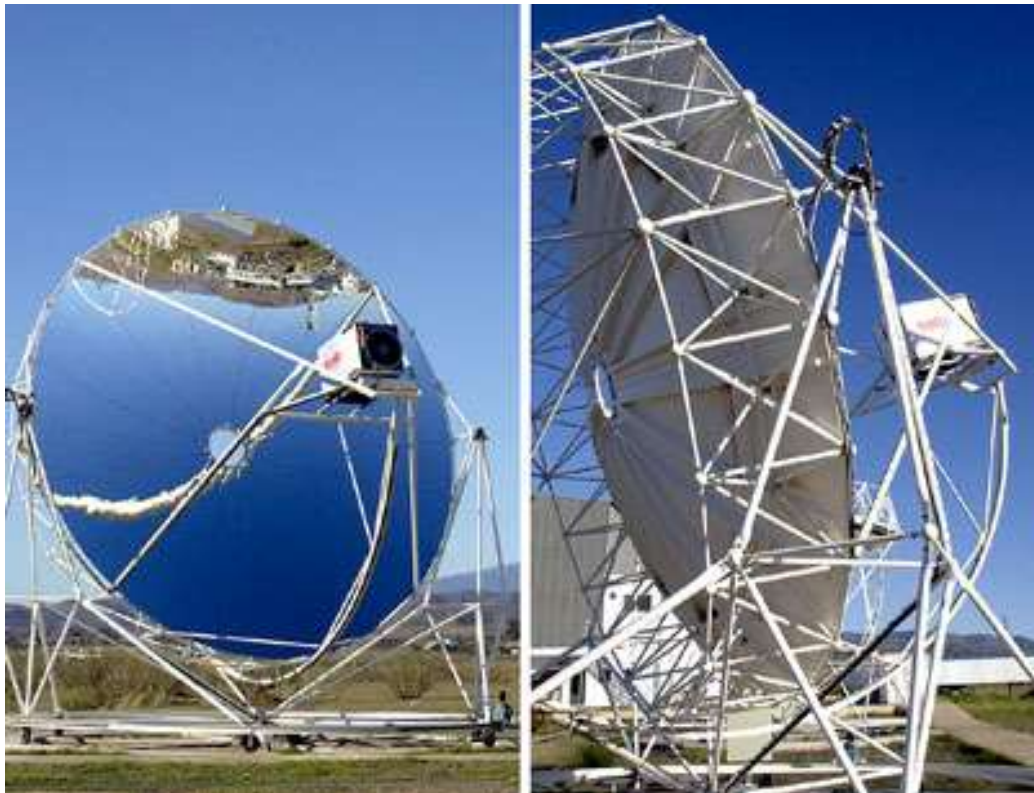
Figure I.6 A parabolic dish at the Plataforma Solar de Almería near Tabernas, Spain (EURODISH, 10 kW).
