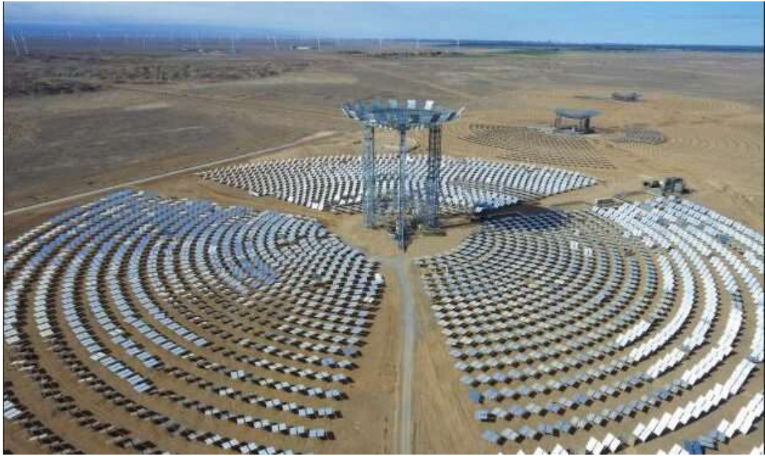
Figure I.5 A beam-down concentrator under construction in the Jiquan prefecture, PRC (Yumen Xinneng, 50 MW).
