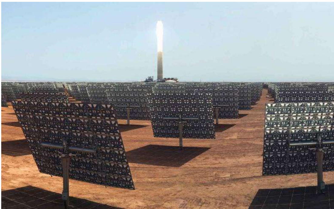
Figure I.4 A central tower receiver in Ouarzazate, Morocco (NOOR III, 150 MW).
