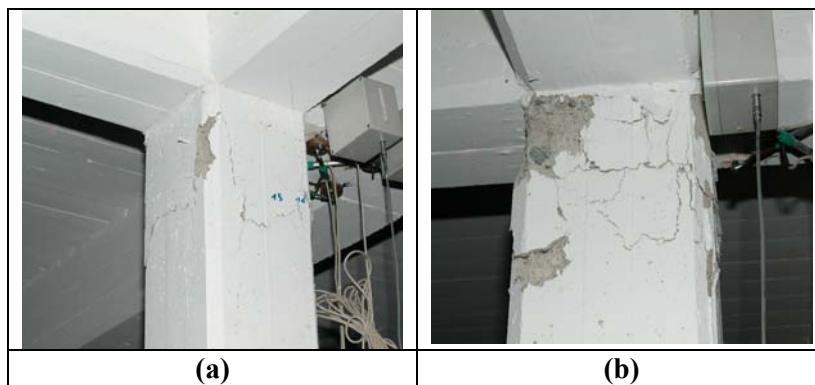
Figure 2.1.2-1 - Damages on column C3 at 1 st floor (a) and 2 nd floor (b)
