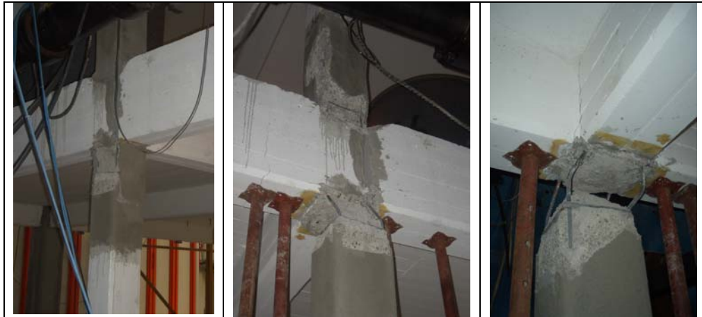
Figure 5.3.2-2 – Column C9 progressive damage.
