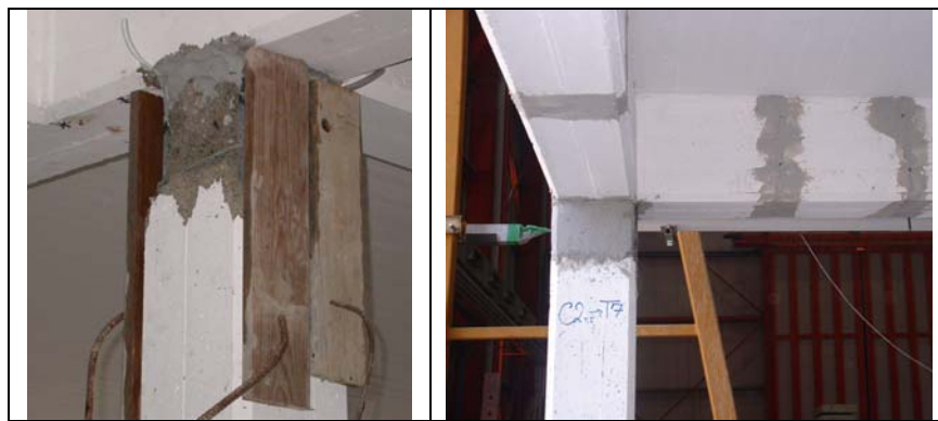
Figure 4.3-1 – Original cross section restoration (a) and injection of cracks
