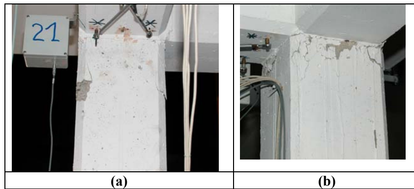
Figure 2.1.2-2 – Damages on column C4 at 1 st floor (a) and 2 nd floor (b)
