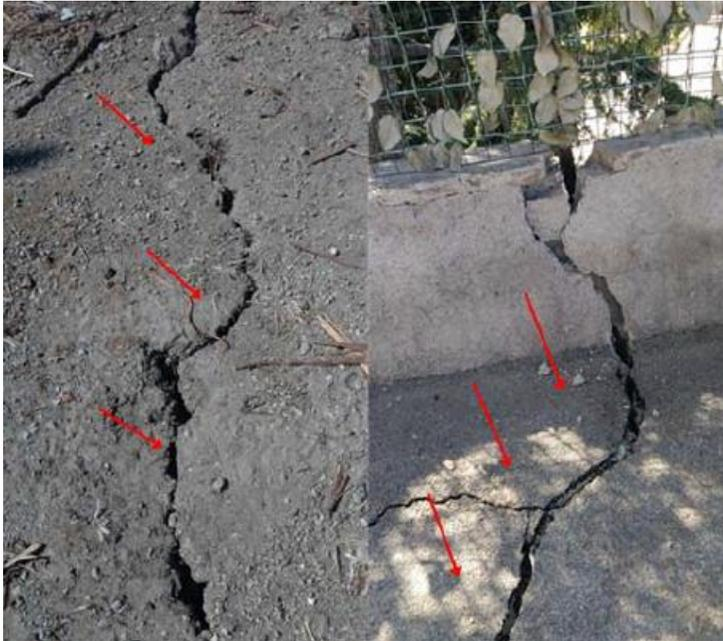
**Figure 5-61:** Example of coseismic ruptures on Crateca road (from Nappi et al. 2017).
