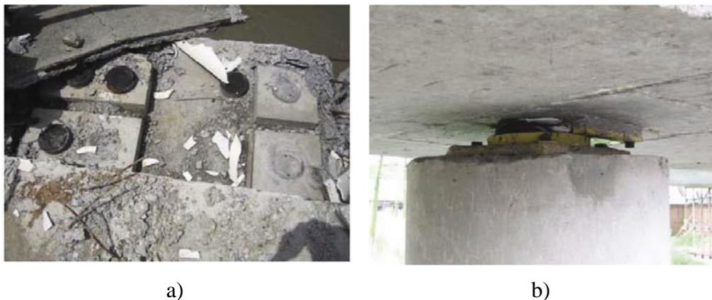
**Figure 12.** Bridge bearings damage in Wenchuan earthquake: (a) Longwei Bridge, (b) Huilan ramp Bridge (Han et al. 2009)
