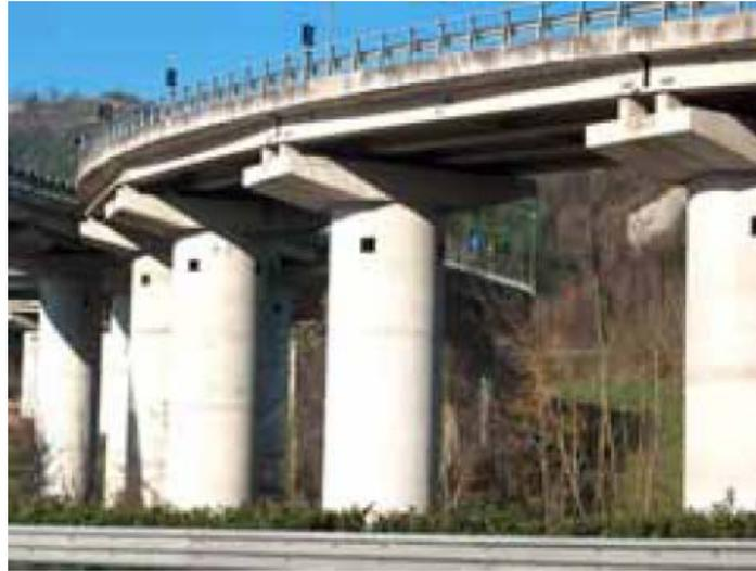
*Figure 1.1 – Hollow Circular Piers (Viaduct Sarsina, Italy)*
