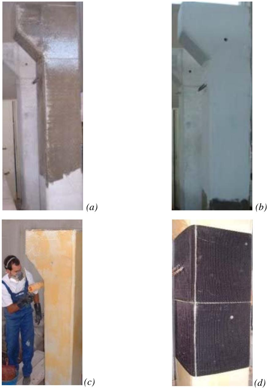
*Figure 2.11 –Strengthening Application: (a) Primer application, (b) putty application, (c) saturating resin application, (d) fabrics application*
