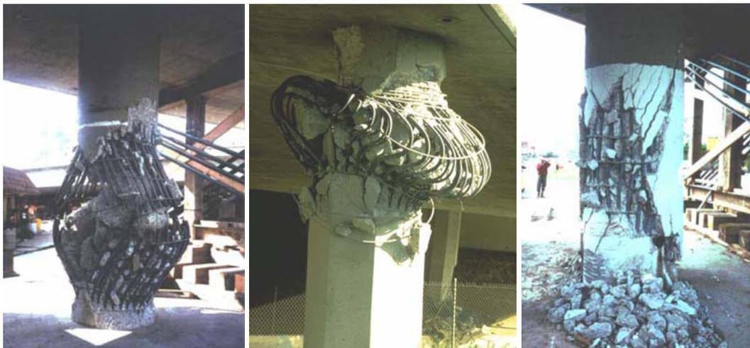
*Figure 1.9 - Different damage patterns for RC piers: symmetric buckling (left) flexural failure (middle) shear failure (right).*
