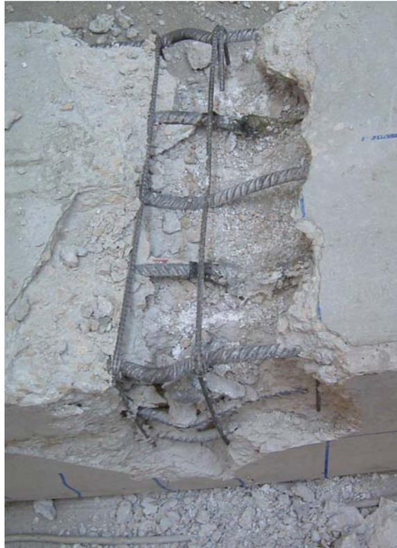
*Figure 4.4 –Crashed concrete removed and steel cage exposed (U2)*
