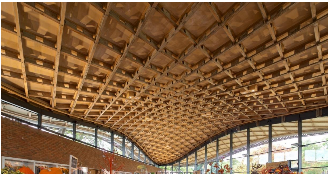
Fig. 6 Savill Garden Building Gridshell, G. Howells
