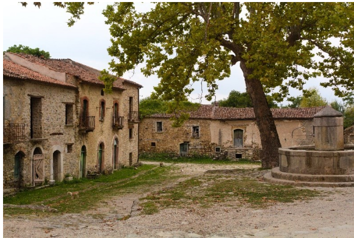
Figure 8 A view of the central square of the old village of Roscigno.
