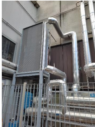
Figure 4.6 Dry cooler of the HVFPCs field thermal block: (a) picture of the dry cooler installed at ground level ; (b) schematic representation of the dry cooler and its circuit.
