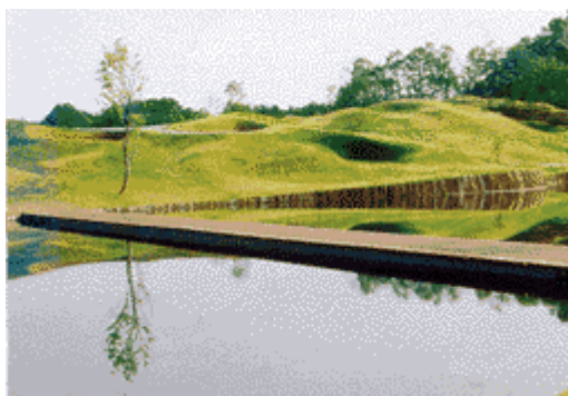
Figure 4 - Use of FRP Tendons in the Pontoon Bridge at Takahiko Three Country Club, Japan
