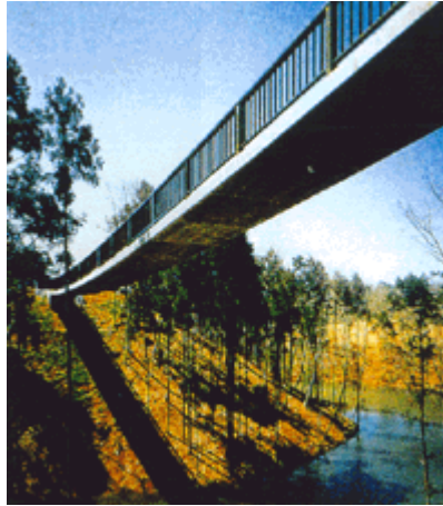
Figure 6 - Use of CFRP Bars in a Stress Ribbon Bridge at the Southern Yard Country Club, Japan
