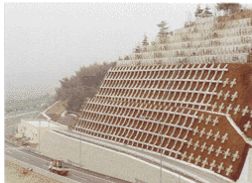
Figure 7 - Use of Technora Elements as Ground Anchors along the Meishin Expressway, Japan
