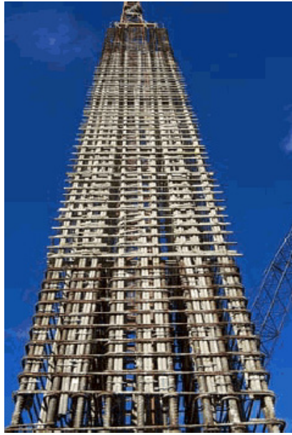
Figure 12 - Tunnelling Boring Application, Bangkok MRTA – Thailand (courtesy: http://www.fortius.be )
