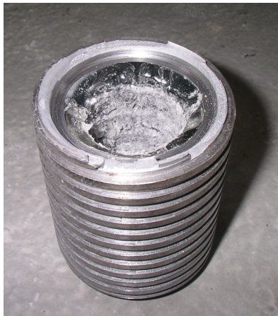
a) Rupture of steel hollow cylinder used as anchoring device
