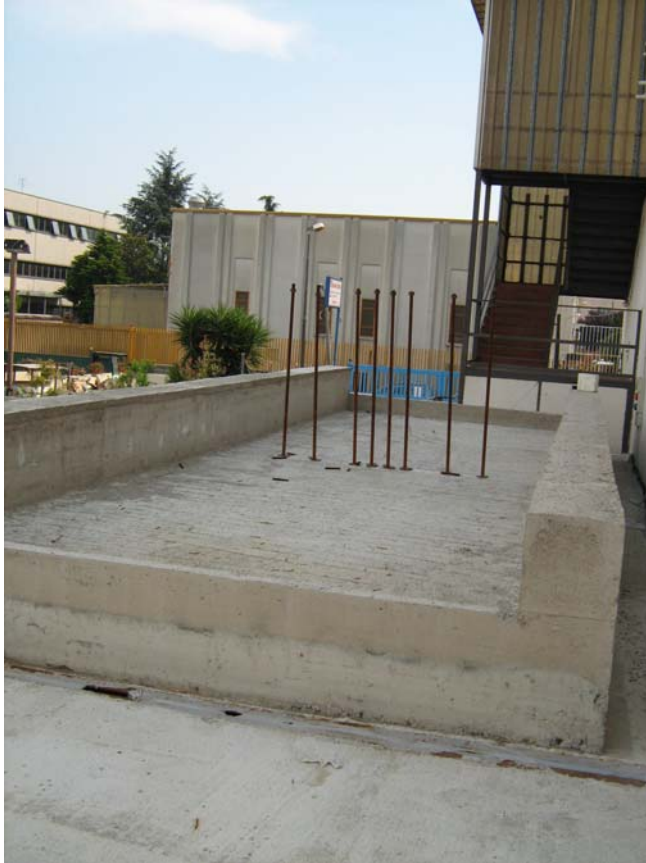
figure 24 concrete slab: the basement
