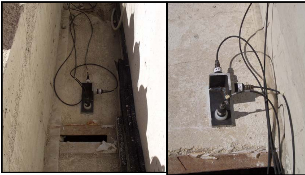
figure 40 accelerometers pos 6-8 and pos 9-11
