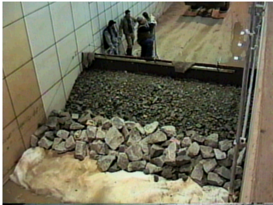
Figure 4.5. Structure installation with an impermeable sheet in the middle
