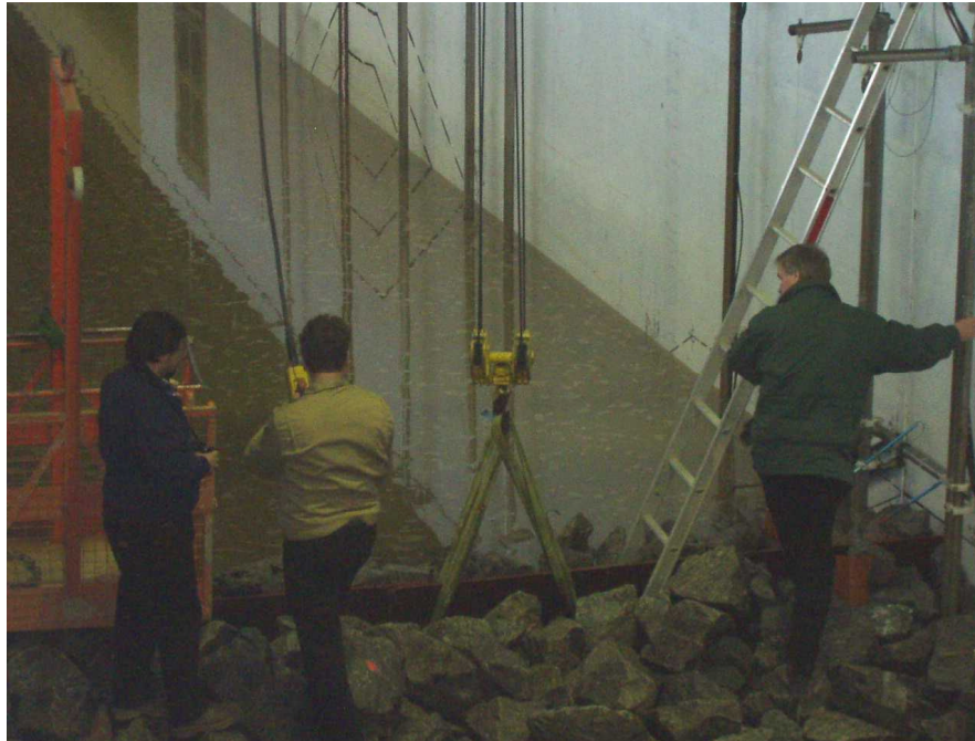
Figure 4.6. Removal of impermeable sheet from middle of structure
