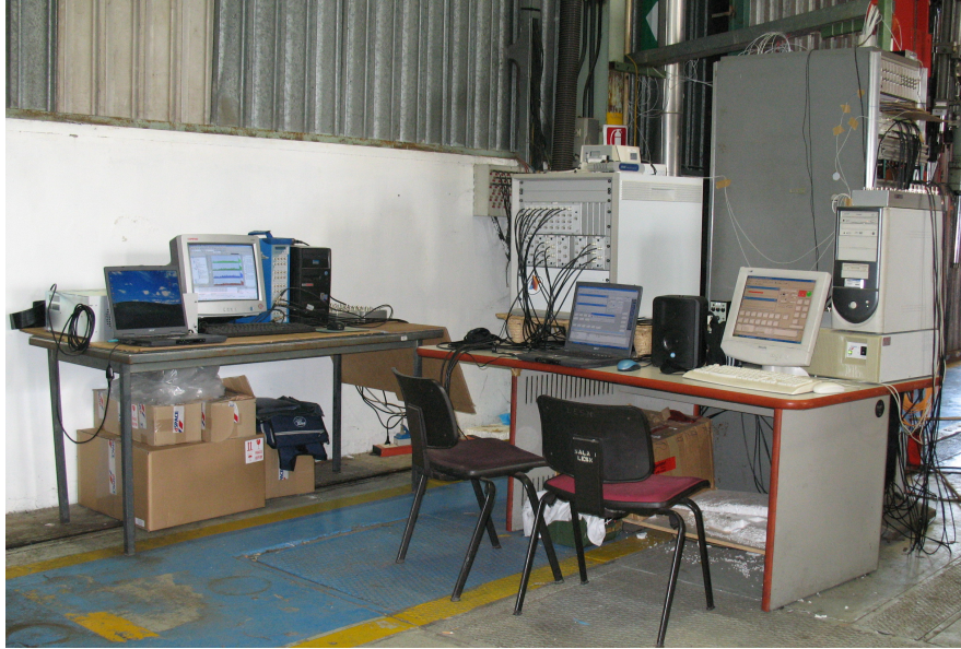
Figure 4-9: View of whole control system
