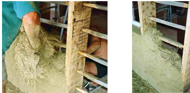
Fig. 11 Messa in opera del torchis (on line: http://www.freewebs.com/torchis/posedutorchis.htm )
