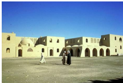
Fig. 34 Villaggio di New Gurna, Hassan Fathy (on line: http://archnet.org/library/images/one-image.tcl?location_id=1547&image_id=16304&start=19&limit=9 )
