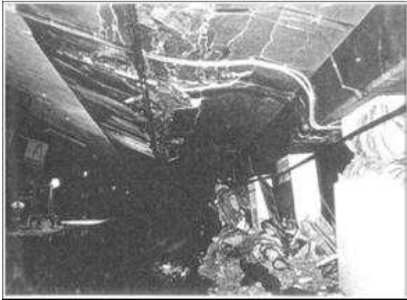
Fig.1.2a: Damage to the Daikai Station during the Kobe earthquake (1995) (Yoshida, 1999)
