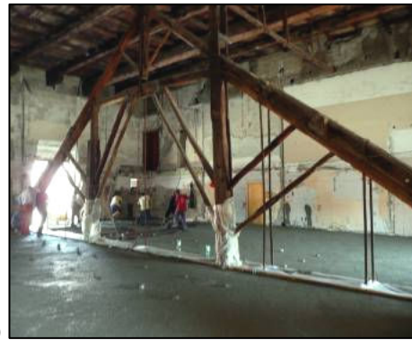
Figure 2.21. Diplomatic Hall (II) – Retrofitting interventions – R.c. slab: a) Before the cast; b) During the cast; c) After the cast.
