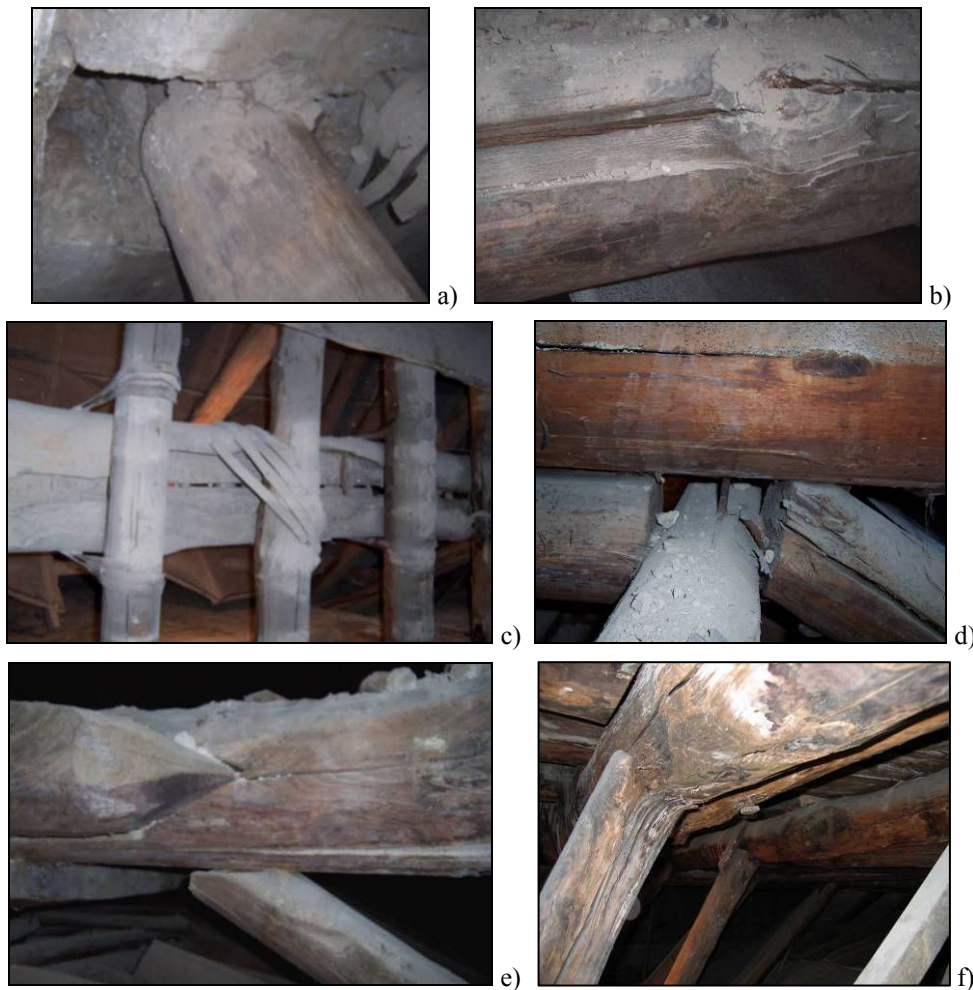
Figure 2.14. Diplomatic Hall (II) – Failure diagnosis: a) Beam support; b) Ring shakes; c) Beam 1A damage; d) Disconnection among elements; e) Beam 5A collapse for bending overstress; f) Strut crushing for compression overstress.
