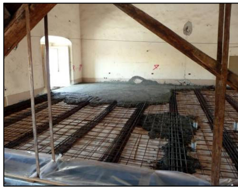
Figure 2.21. Diplomatic Hall (II) – Retrofitting interventions – R.c. slab: a) Before the cast; b) During the cast; c) After the cast.
