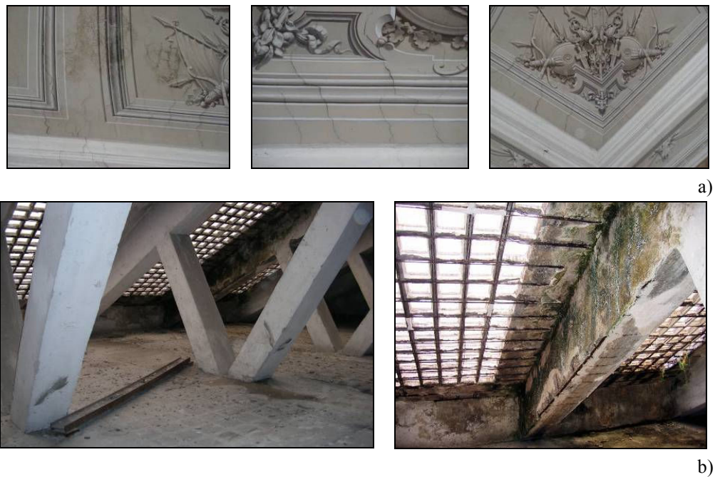
Figure 2.48. Guard Room (XXIX) – Failure diagnosis: a) Humidity spots and fissures of the fresco at the intrados of the vault; b) Damage of r.c. roof.
