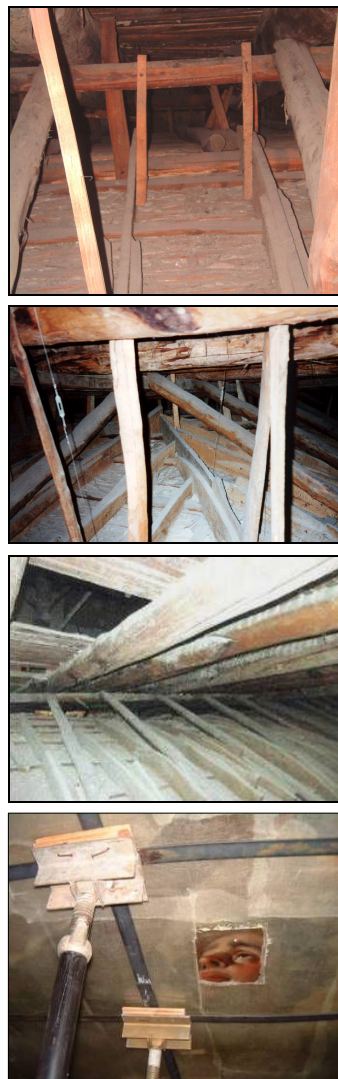
Figure 2.11. Diplomatic Hall (II) – Geometrical survey – Vault structure: a) Carpentry and structural sections [m]; b) Photographic survey.
