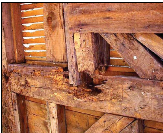
Figure 1.8. Biodeterioration of wood: rotten wood.
