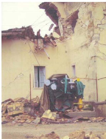
Figure C.3 RG housed in a masonry kiosk closed to building and damaged following the 6 th April 2009 earthquake
