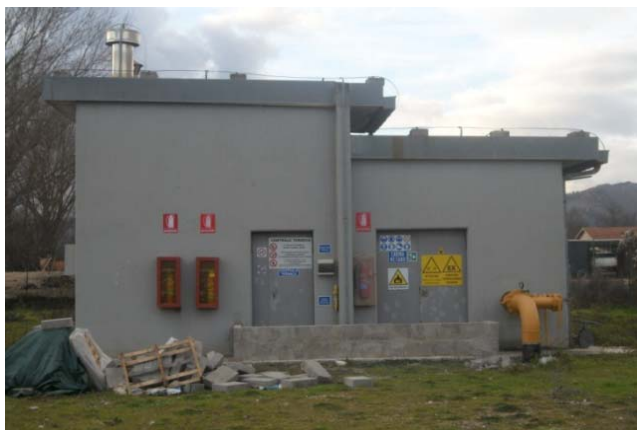
Figure C.2 M/R Metering/Pressure reduction station in Onna (L’Aquila, Italy)
