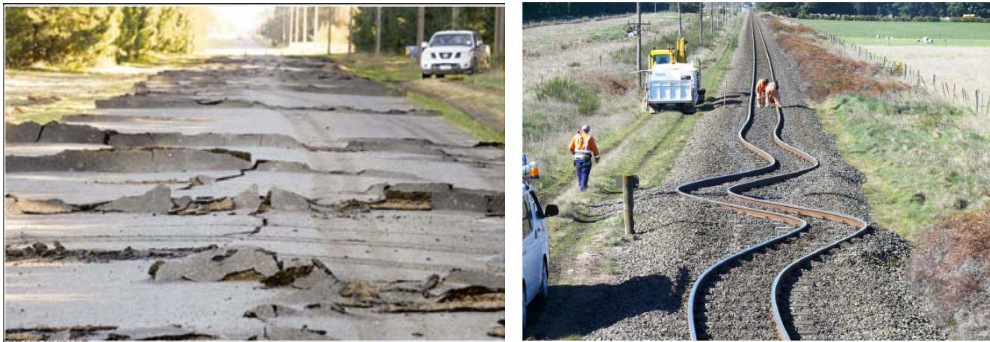
Figure 1.1 Damages on roads (left) and rails (right) due to surface faulting following the 4 September 2010 Mw 7.1 Canterbury, New Zealand Earthquake (Eidinger, 2011)
