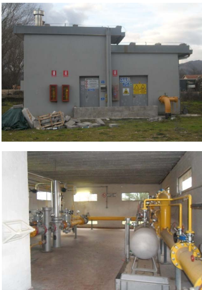
Figure 3.5 Metering/Pressure Reduction Stations external view (up) internal view (down)
