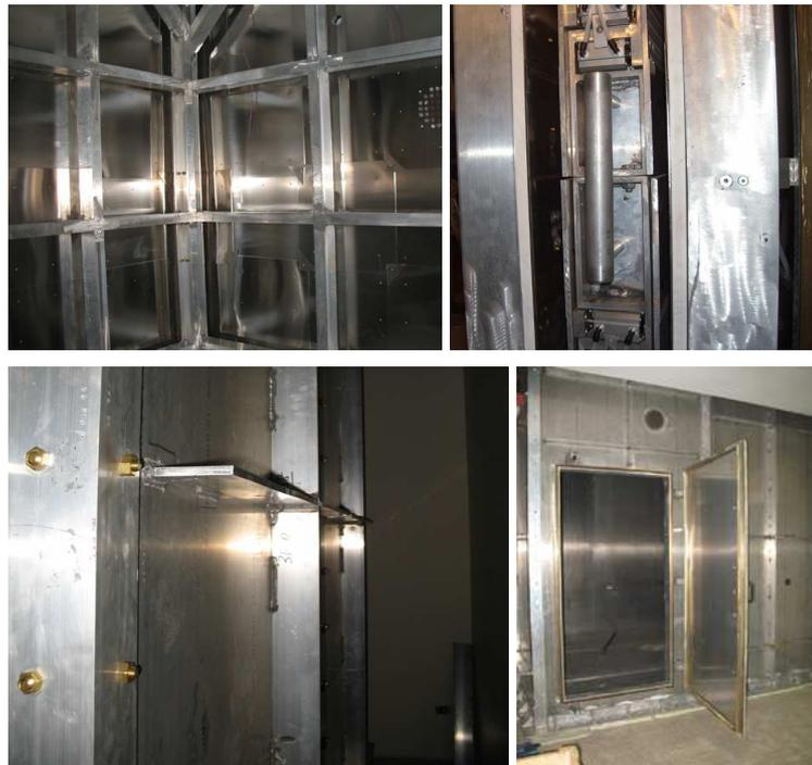
Figure 3.14 – Particular of the shielding room (during the assembling) showing in clockwise direction: The  $\mu$ -metal layer and the aluminum frame structure, the pneumatic door, the external aluminum door and outer aluminum layer.
