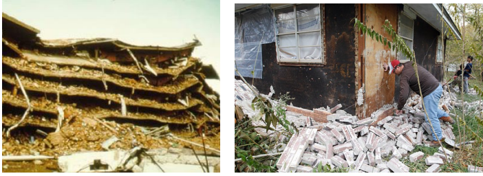
Figure 1.1.: The damage caused by induced earthquakes, left image is showing Collapse of a block of flats in Welkom in 1976 after a mining-related earthquake of magnitude 5.2 (Images courtesy: of the Council for Geoscience, South Africa (SAWDIS)) and the right image is showing a house damaged in a pair of earthquakes that struck Sparks, Oklahoma, Nov. 6, 2011, in less than 24 hours, which is connected fracking while shale gas extraction (By : Bryan Walsh is a senior writer at TIME).
