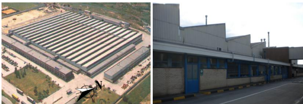
Figure 6.1 Aerial (left) and close-up (right) view of the whole facility
