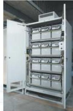
**Figure 2.31 – Composition of CAPAPOST regenerative power storage system [107]**
