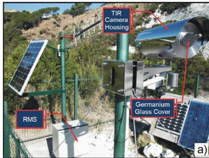
Figure 4.16: Solfatara thermal monitoring station [from Chiodini et al., 2007].
