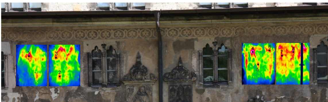
Fig. 3.23: Thermal images that overlap the investigated structure. The numbers indicate the modeled anomalies.
